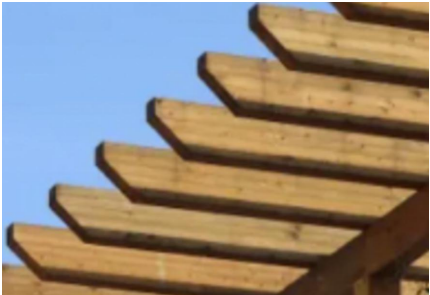
MATERIAL 7: TIMBER PERGOLAS
