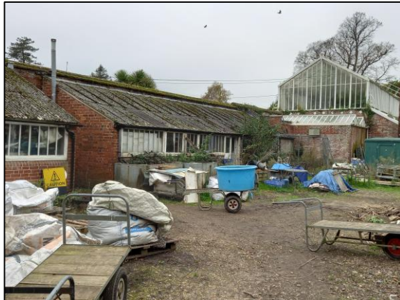
Photo 1 Potting Shed – view from north-east
