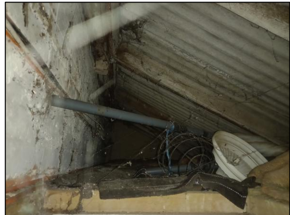
Photo 4 Room 61, interior of roof cavity
