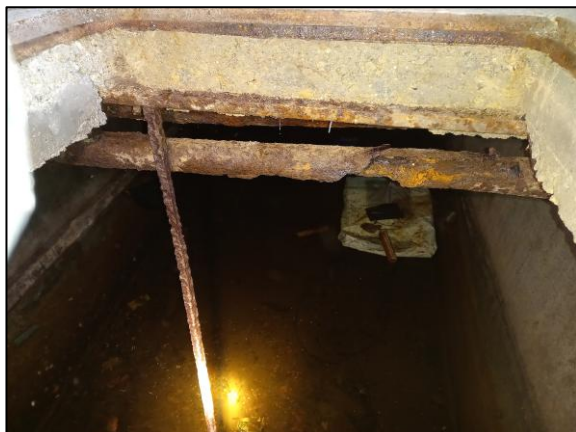
Photo 5 Room 61 – view into tanked cellar with water storage
