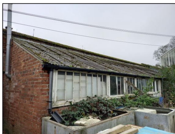
Photo 12 General view of Potting Shed externals
