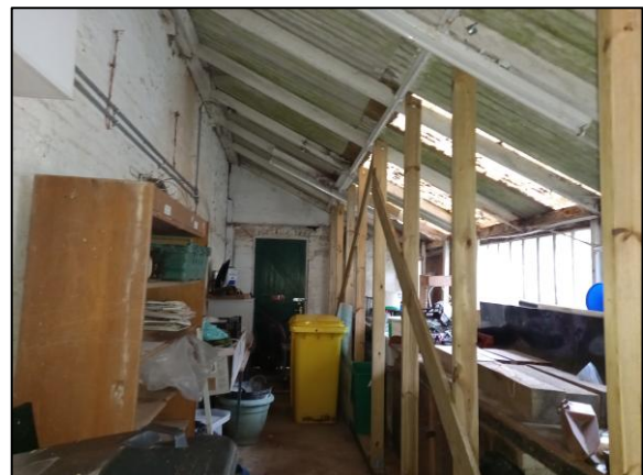
Photo 6 Room 62, view towards west
