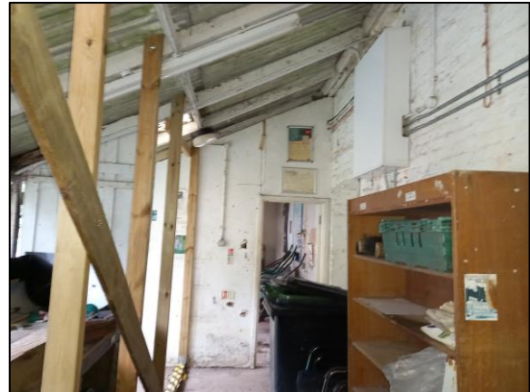
Photo 2 View from west to east showing partition wall
