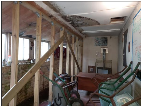
Photo 3 Room 61 view east showing boarded ceiling and hatch
