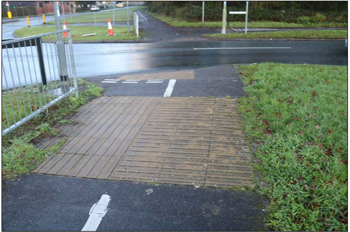
Figure 2.11 Crossing Infrastructure on Wakeford Way
