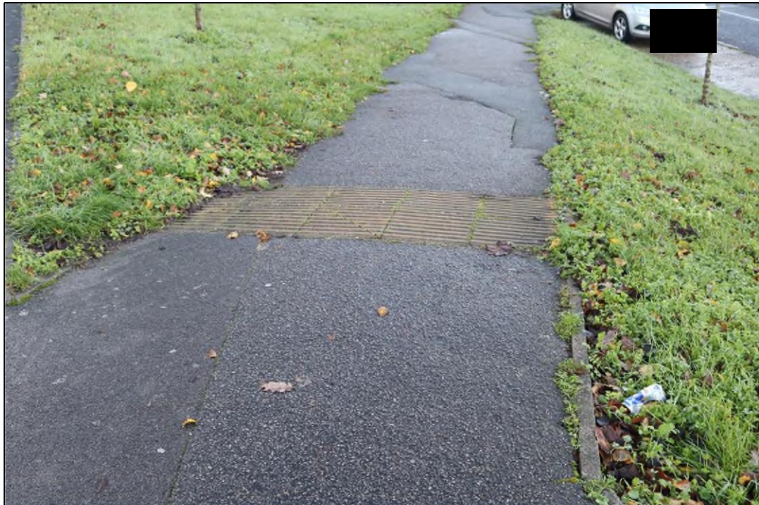
Figure 2.3: Corduroy Paving
