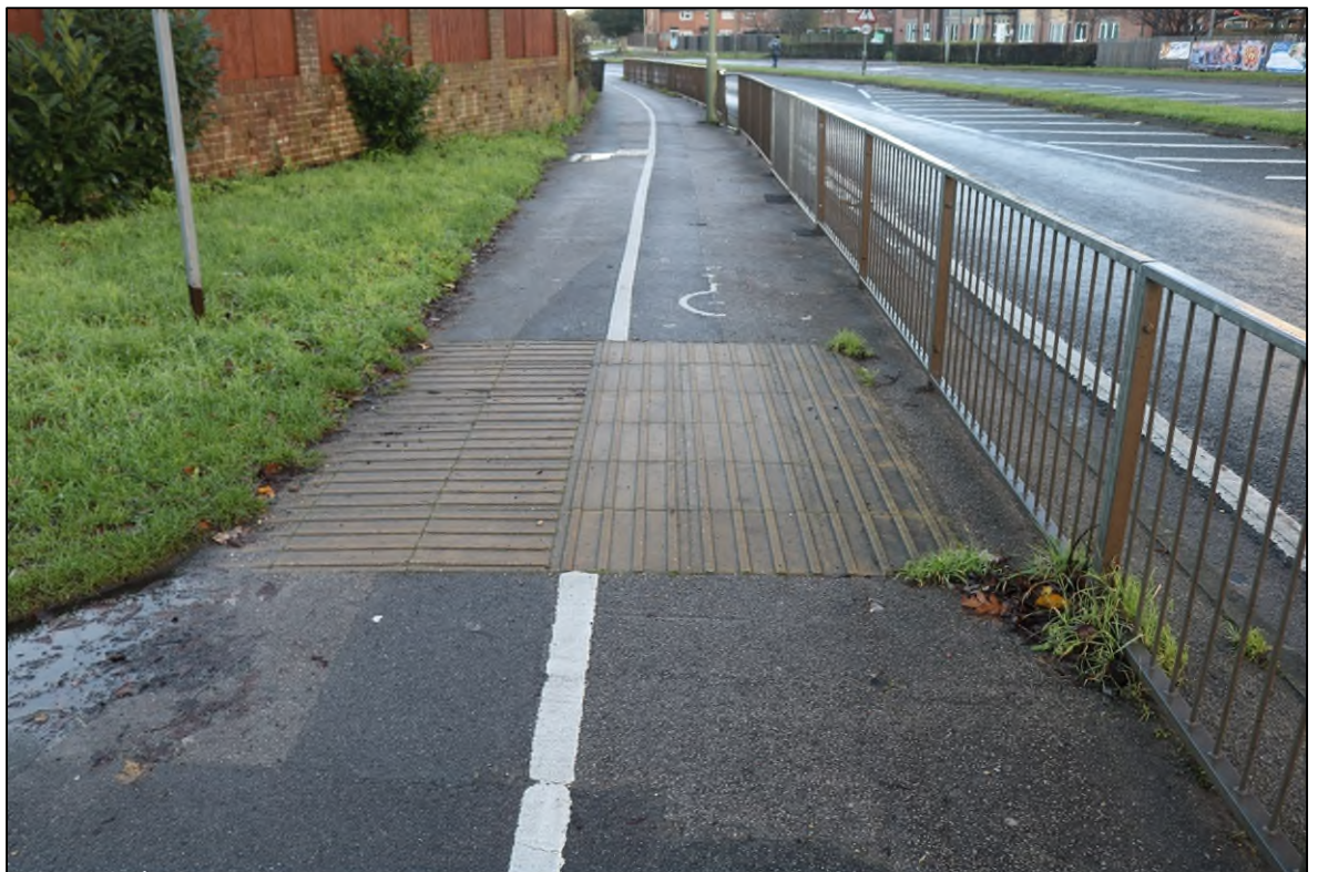
Figure 2.16: White Lining and Corduroy Paving
