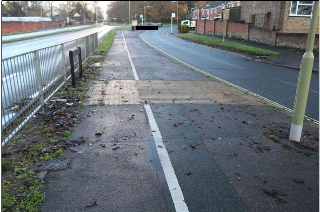
Figure 2.9 Corduroy Paving and Railings
