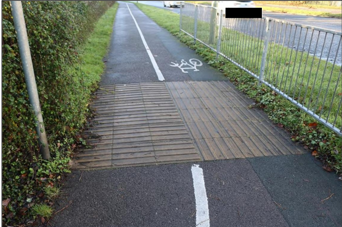
Figure 2.14: Shared footway/cycleway along Petersfield Road
