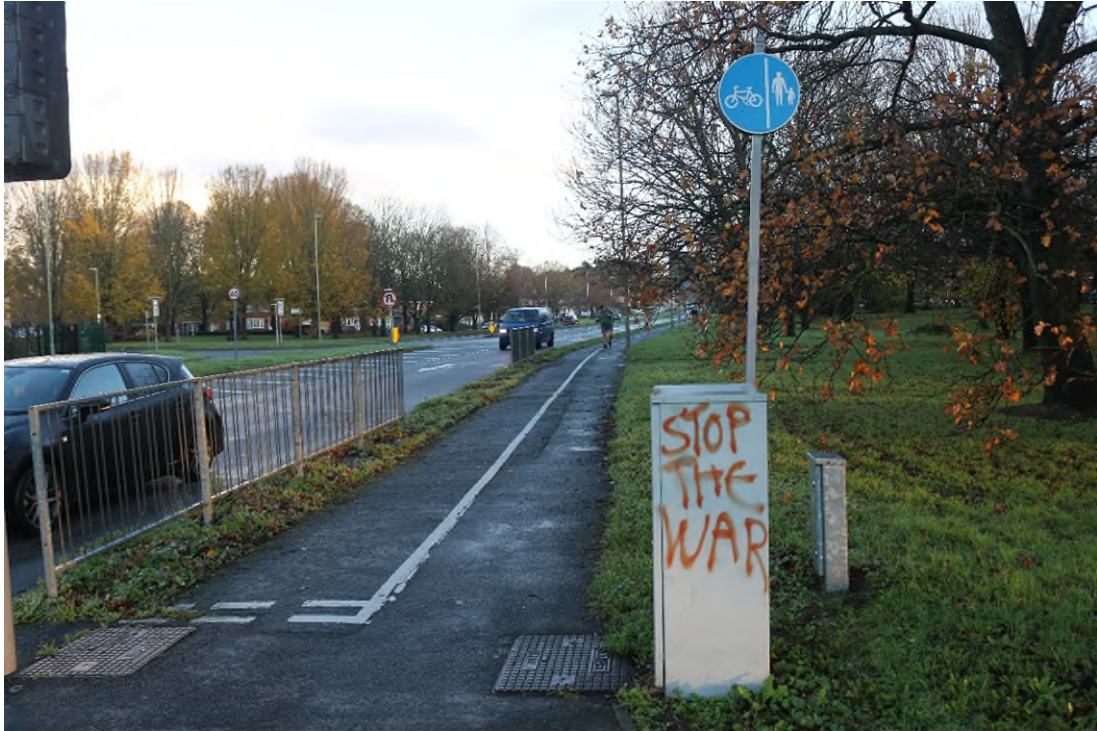
Figure 2.36: Shared Footway/Cycle along East Side of Petersfield Road
