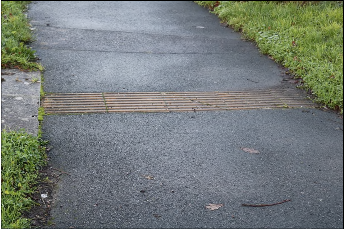
Figure 2.15: Well -maintained Tactile Paving
