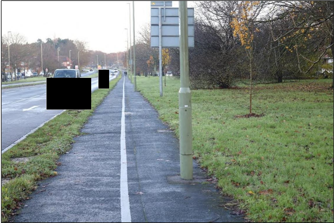
Figure 2.6: Localised Surfacing repairs
