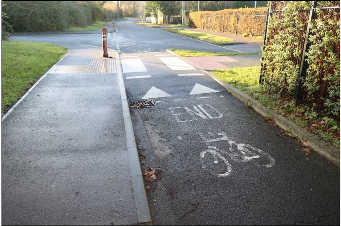
Figure 2.23: Raised table at crossing point
