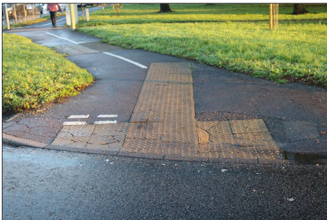
Figure 2.2: Tactile Paving at access from Bartons Road
