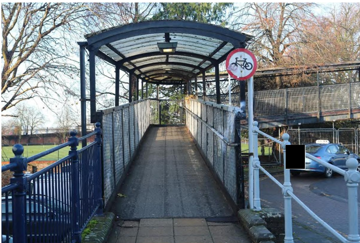
Figure 2.28: Railway Footbridge and Ramp
