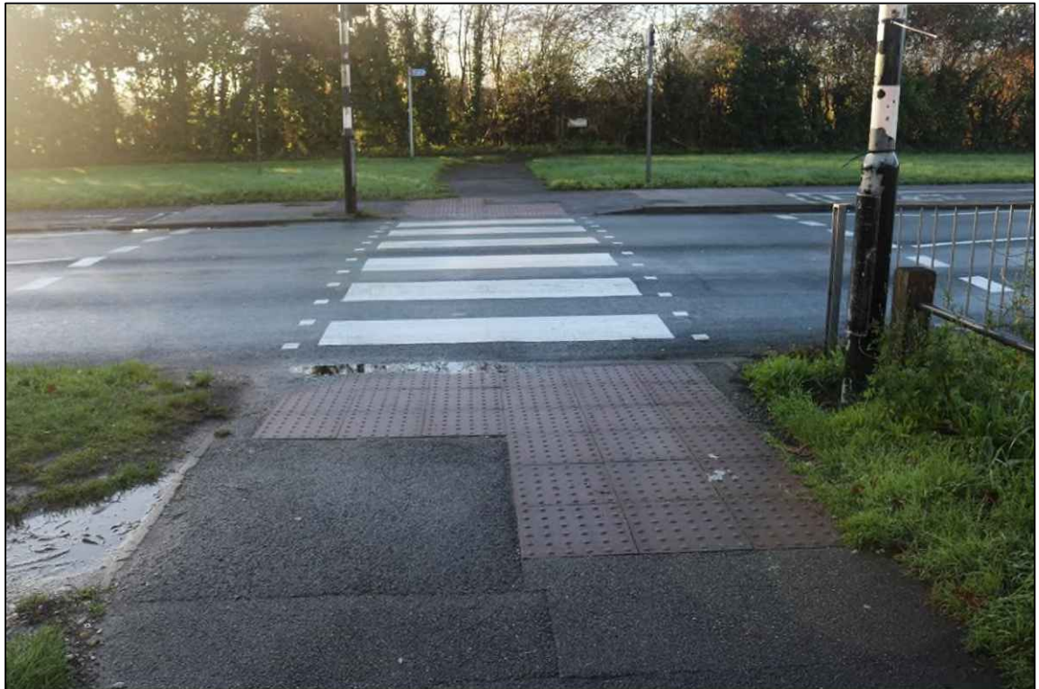
Figure 2.21: Well-Maintained Crossing Point
