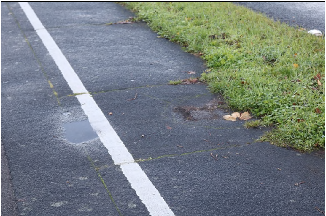
Figure 2.6: Localised Surfacing repairs
