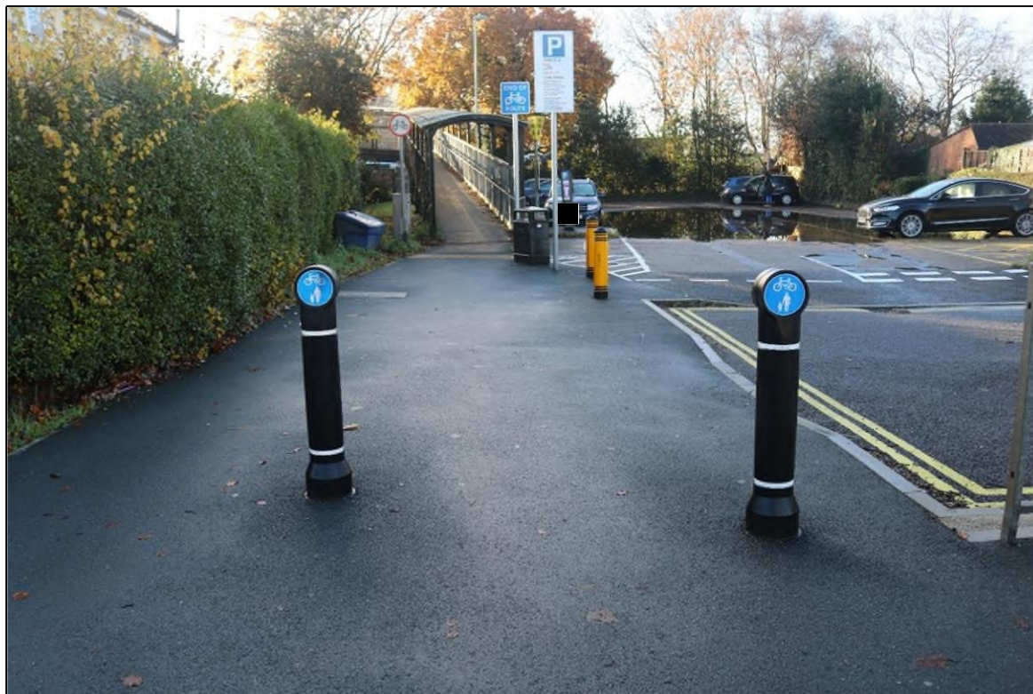
Figure 2.27: Approach to the railway footbridge
