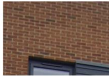
MATERIAL 2: BRICKWORK NEW AND OLD
