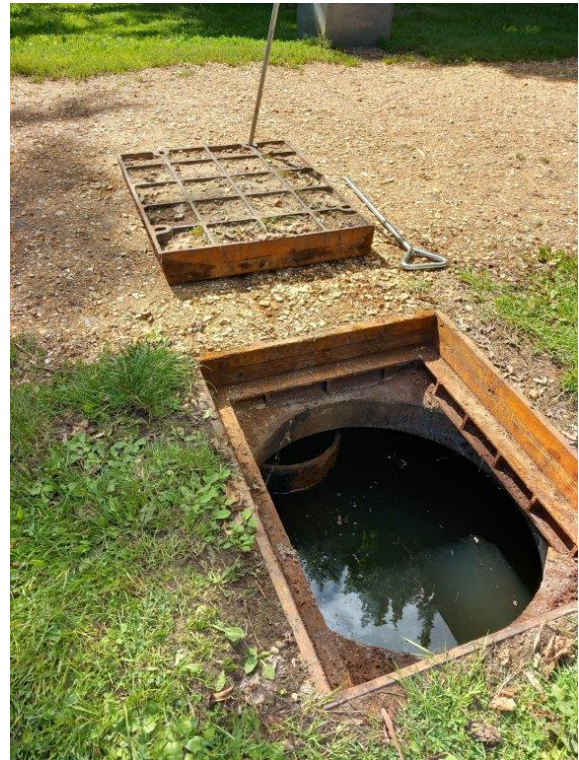
8) 300mm diameter pipe outlet into downstream watercourse, south of lake [Report Section 5.2, f)]
