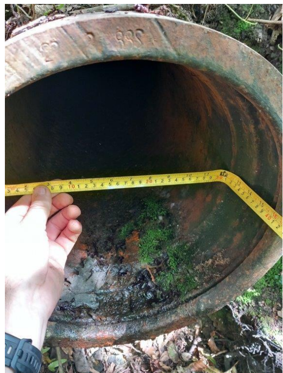
8) 300mm diameter pipe outlet into downstream watercourse, south of lake [Report Section 5.2, f)]
