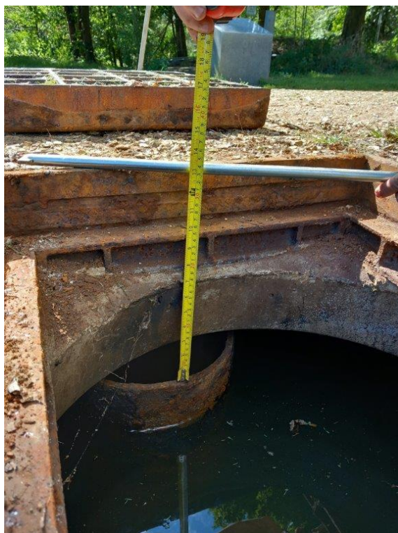
7) On-line outlet pipe weir approximately 0.33m below cover level [Report Section 5.2, e)]
