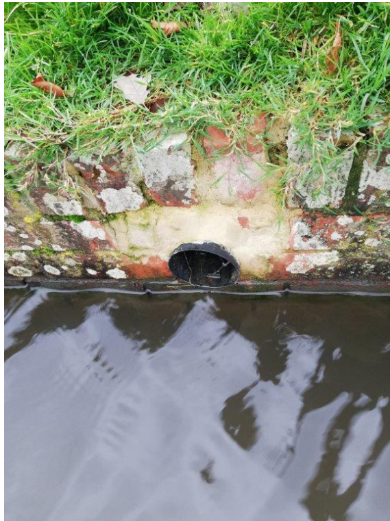
7) On-line outlet pipe weir approximately 0.33m below cover level [Report Section 5.2, e)]
