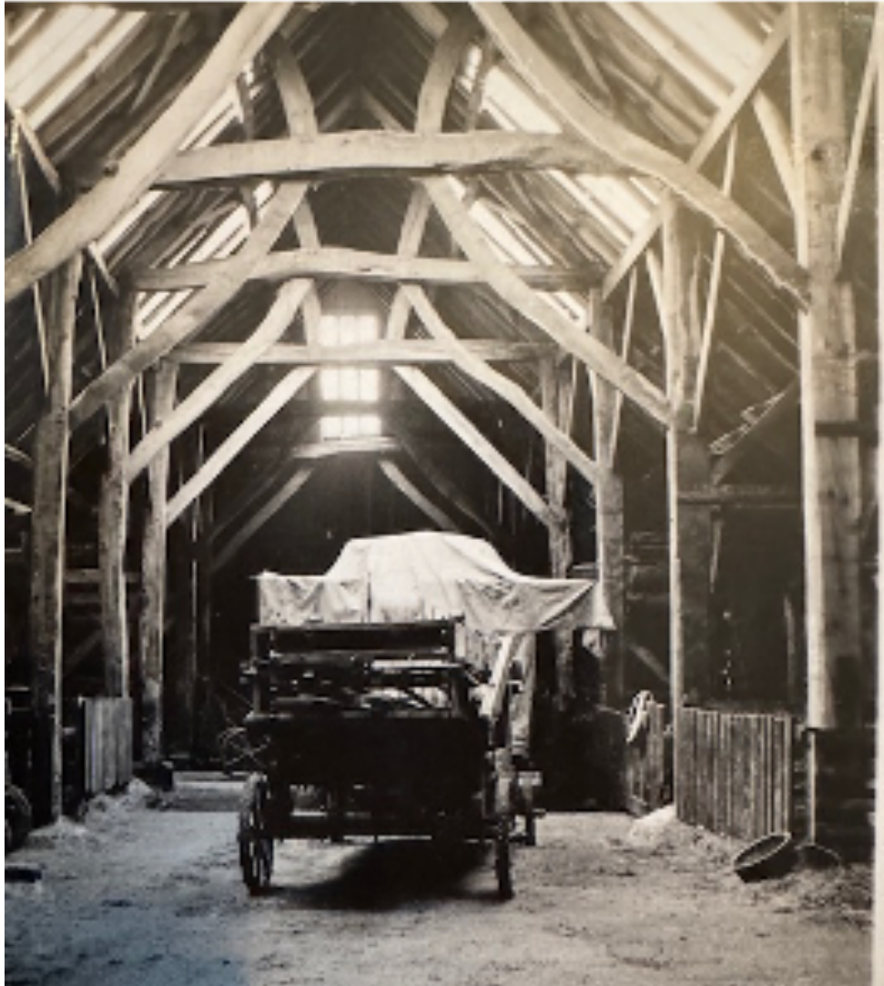
The barn with a corrugated roof and windows along both roof slopes as well as in the gable end.
