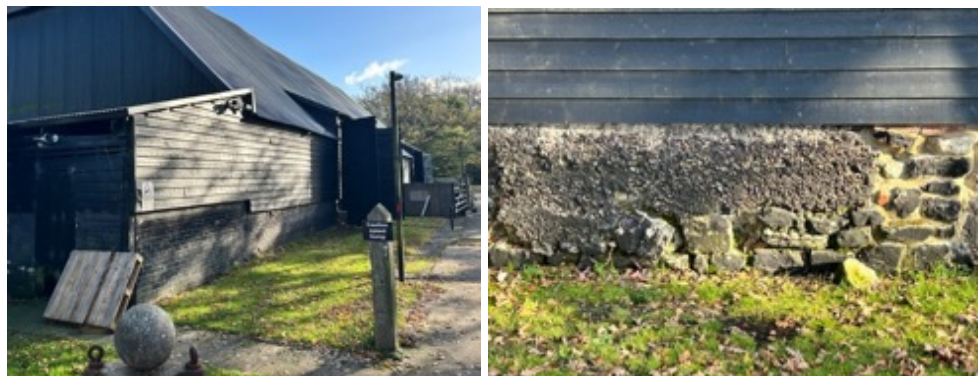
The northwest corner wall replaced in brick and a concrete repair.
