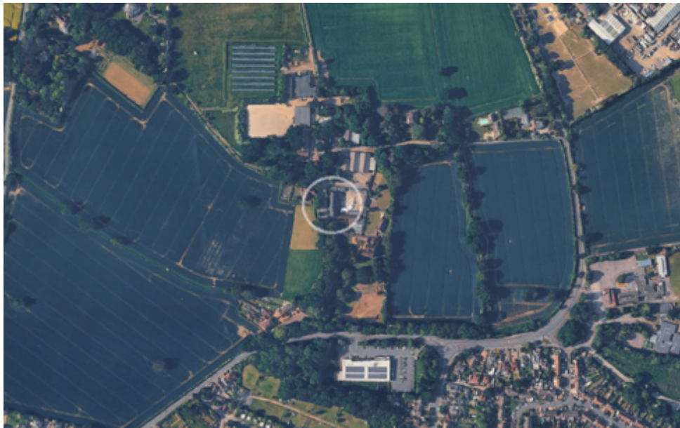
Aerial view of the barn at Manor Farm, highlighted. © Google
