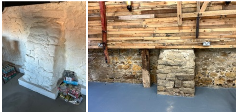
Remnants of the buttressing in the east and north walls.
