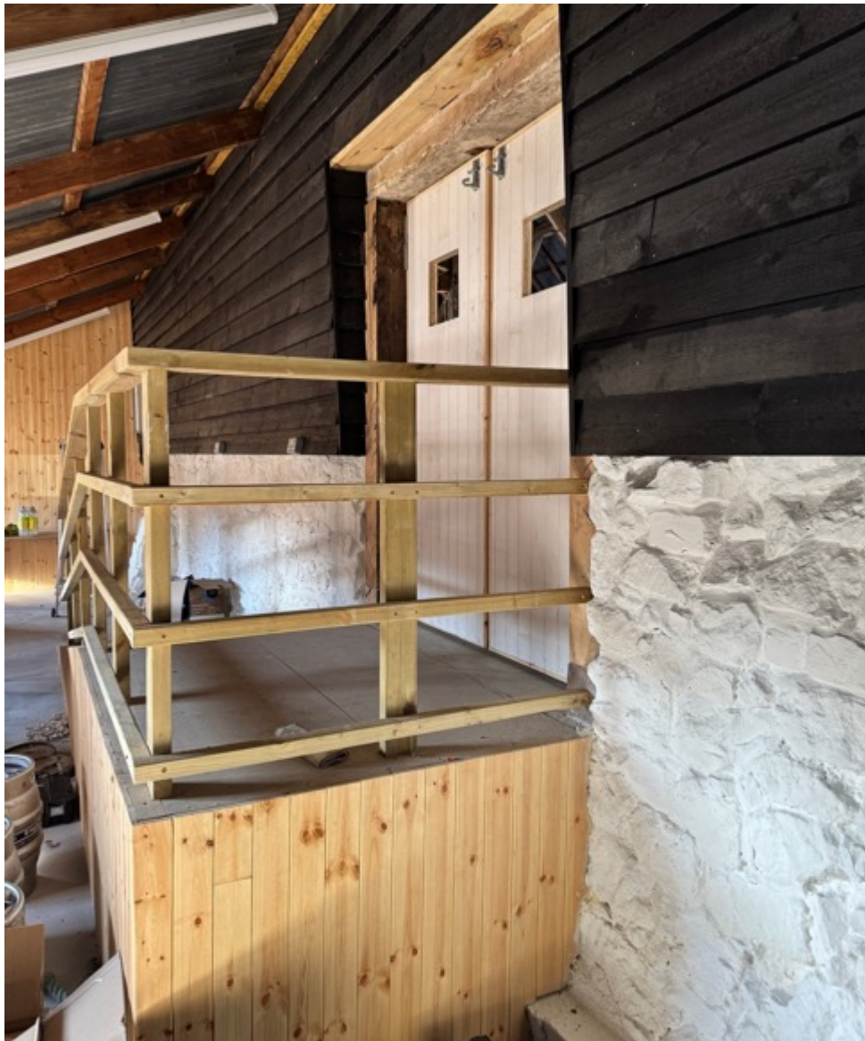
The doors and ramp view from within the extension to the east.
