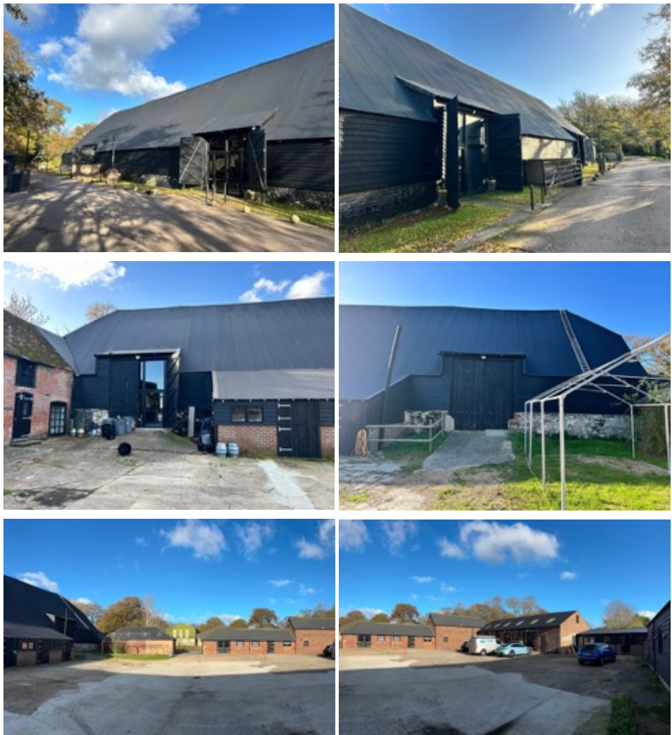
The west and east elevations of the barn and courtyard viewed from the south.
