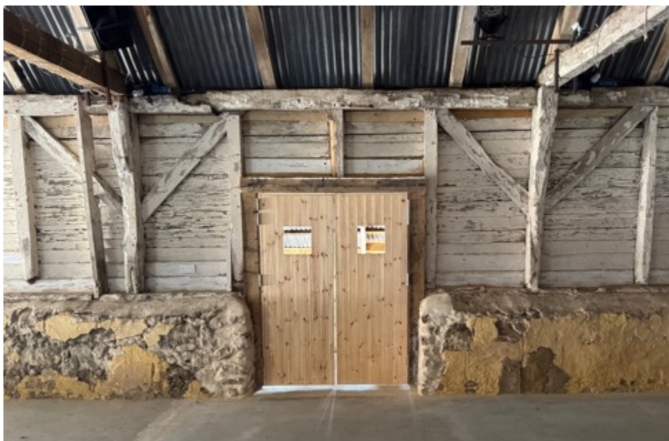
The doors as implemented and seen from within the barn.
