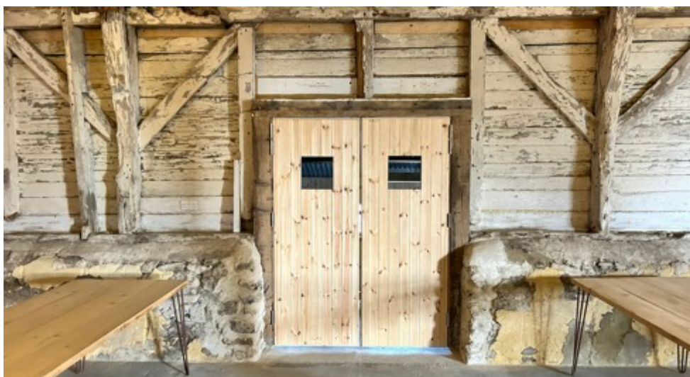
The new opening which connects the barn with the extension to the east.
