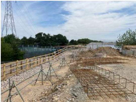
View towards Northeast over Criblock retaining wall to B&Q access road
