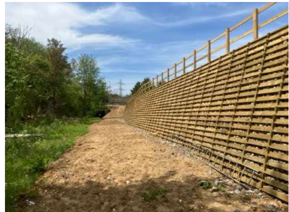
View of southern boundary and retaining wall
