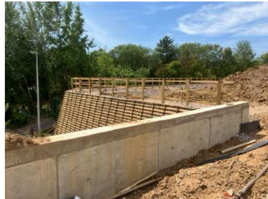
View towards East and B&Q car park of completed retaining walls.
