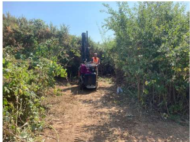
View towards South from the centre of the site at the time of Remada's Ground Investigation
