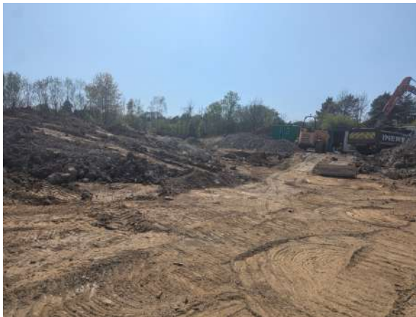
View towards west (site entrance) with reduced level dig in progress
