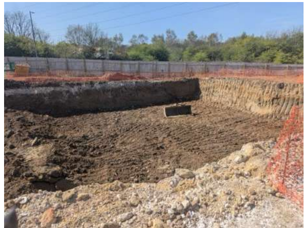
View towards west of attenuation tank excavation
