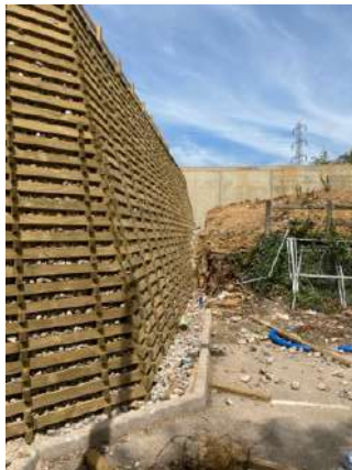
View from B&Q car park of pre-cast and Criblock retaining walls
