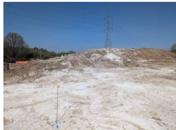
View towards North
