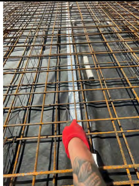
Photograph of mechanical stress point testing being carried out on site.
