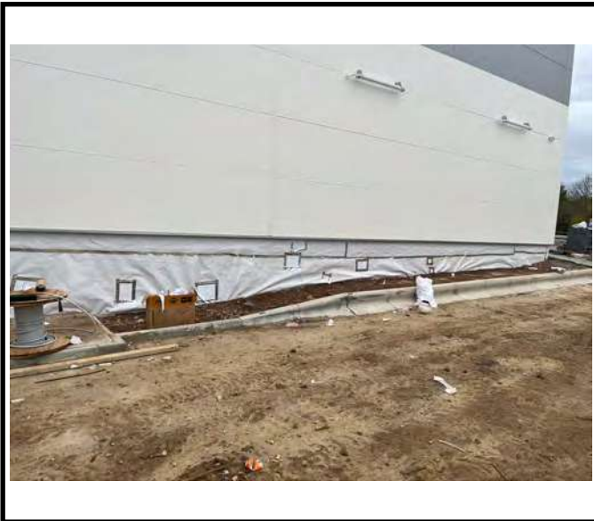
An overview of the completed perimeter detailing.
