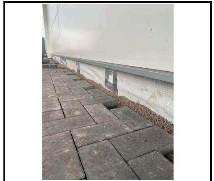
An alternative overview of the completed perimeter detailing.
