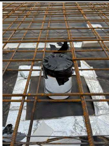
Additional photograph supplied by the client
