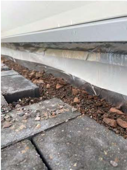
An alternative overview of the completed perimeter detailing.
