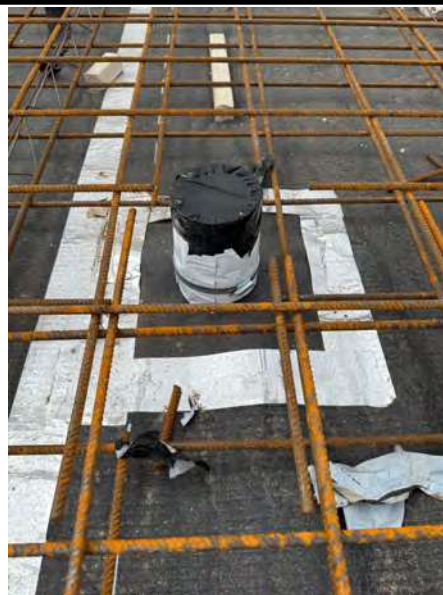
Additional photograph supplied by the client
