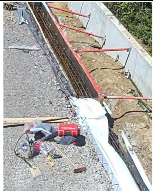
Additional photo of pre poured concrete perimeter sections
