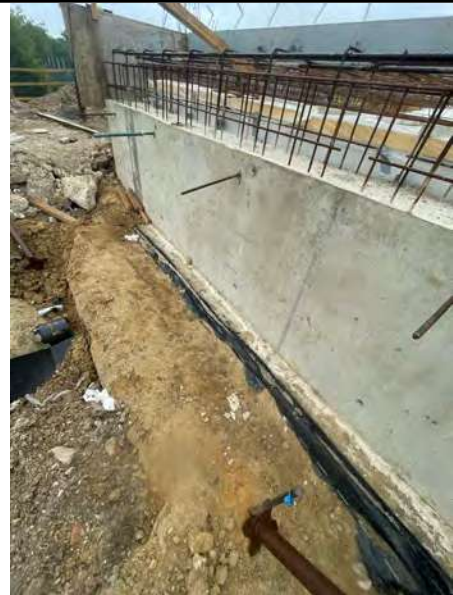
Additional photo of per poured concrete perimeter sections
