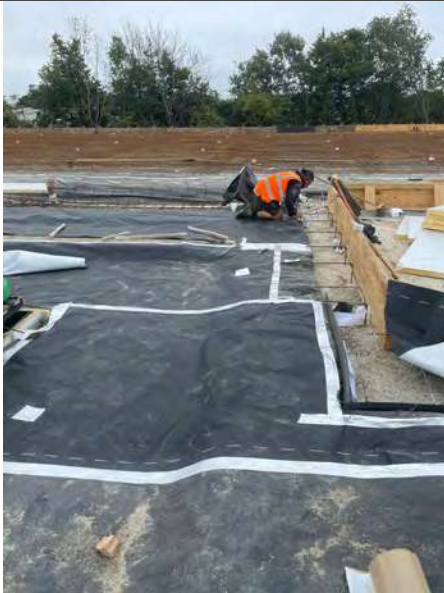
Photo of the installation team carrying out the installation
