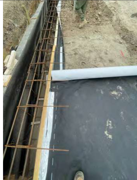
Additional photo of the install progressing
