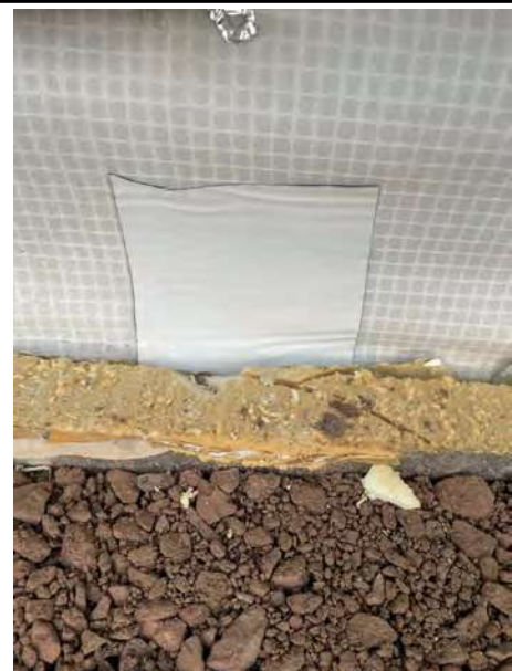
A hole in the membrane that has been repaired using a patch of Cordex EPS GRM.
