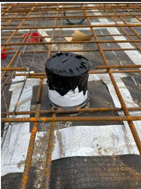
Additional photograph supplied by the client
