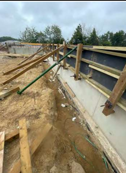
Additional photo of per poured concrete perimeter sections
