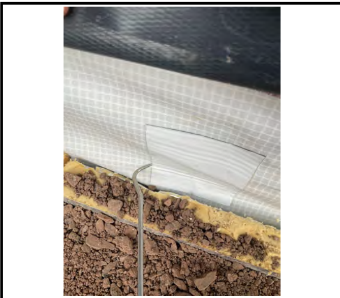
A mechanical point stress test being conducted upon the puncture, repaired using a patch of Corden EPS GRM.
