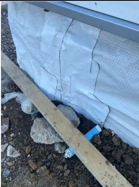
Strips of Corden EPS GRM Self Adhesive Membrane applied around the corner to seal the area.
