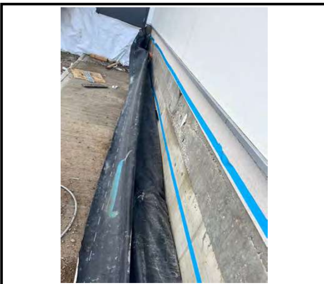
The Corden EPS Double Sided Butyl Tape applied prior to installation of the Corden EPS Total Gas Barrier.
