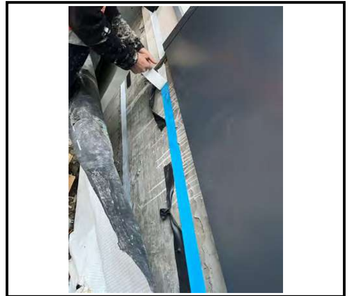
The Corden EPS Double Sided Butyl Tape being applied prior to installation of the Corden EPS Total Gas Barrier.
