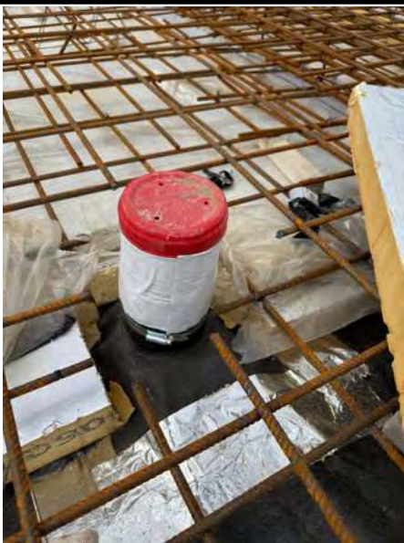
Additional photograph supplied by the client
