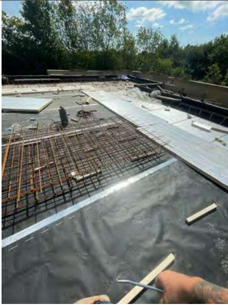
Additional photo of area where verification inspection took place.
