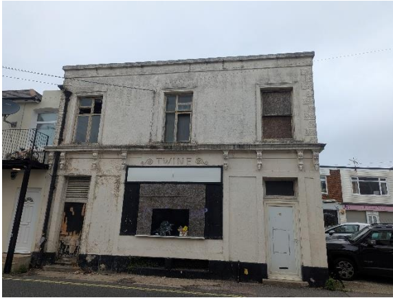
Photo 1 – external view of building 1, south elevation
