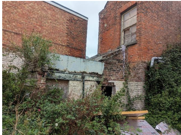
Photo 4 – external view of building 3 – lean-to (east)
