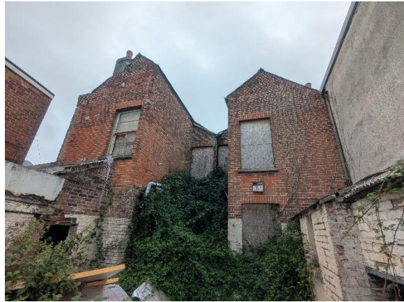
Photo 2 – external view of building 1, north elevation
