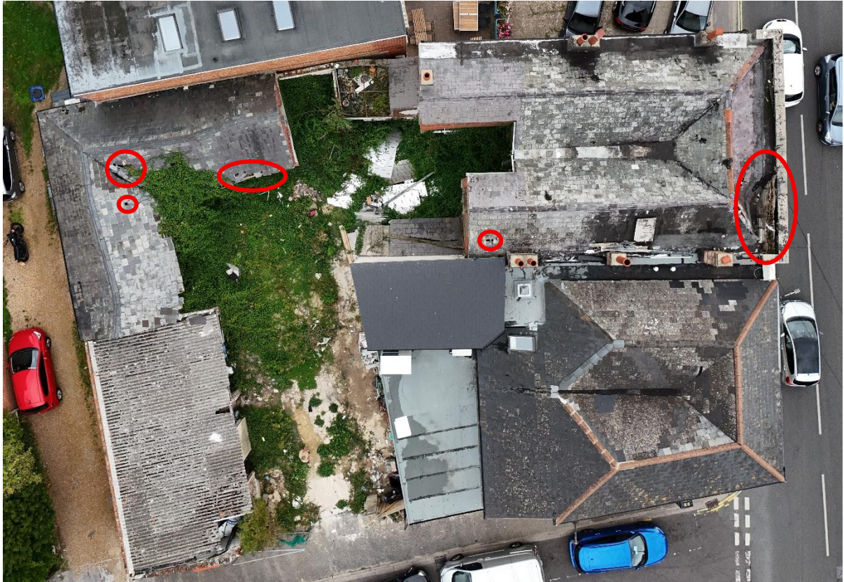
Photo 14 – drone photo of site facing north, showing collapsed roof on building 1
