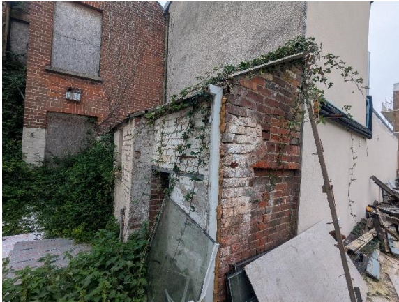
Photo 3 – external view of building 2 – lean-to (west)
