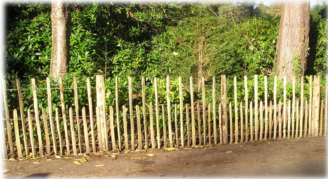
Figure 4: Cleft chestnut paling fencing
