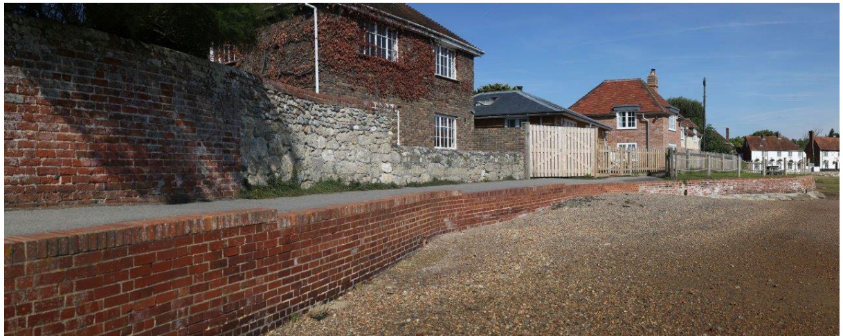
Figure 4.3: View of Langstone High Street
