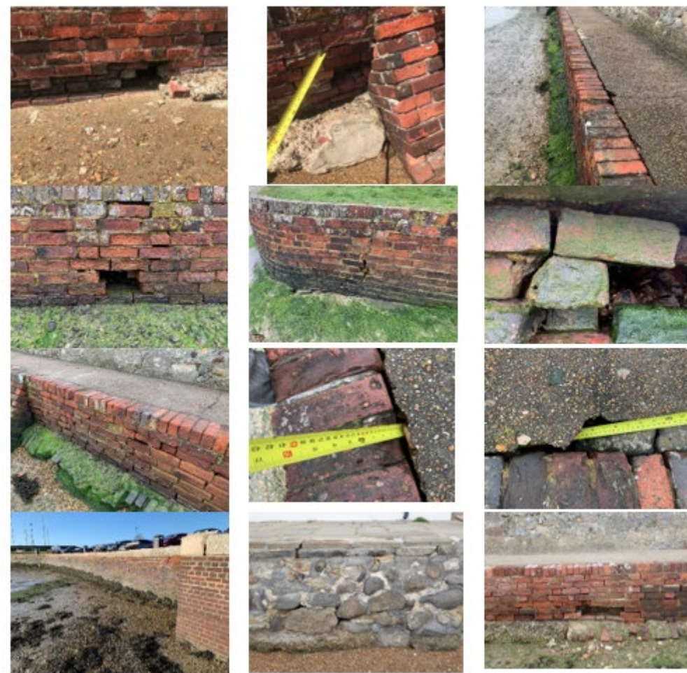
Figure 1.4: Photos showing existing condition of flood defences
