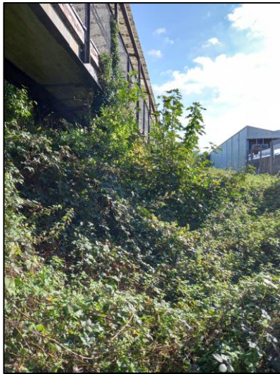
Photo 12 View along railway boundary to west of proposed bridge location.
