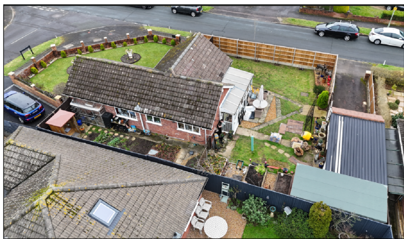
REAR ELEVATION PHOTO
