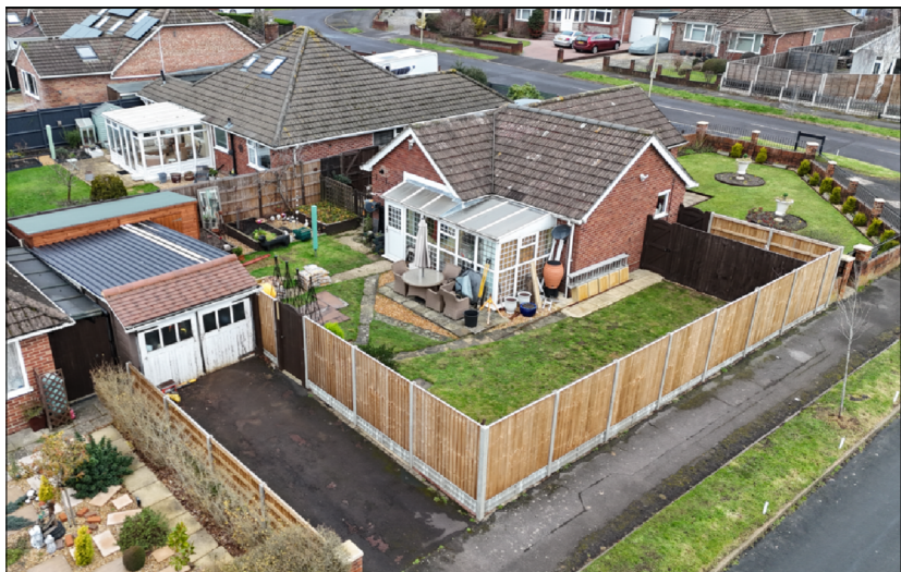
REAR ELEVATION PHOTO
