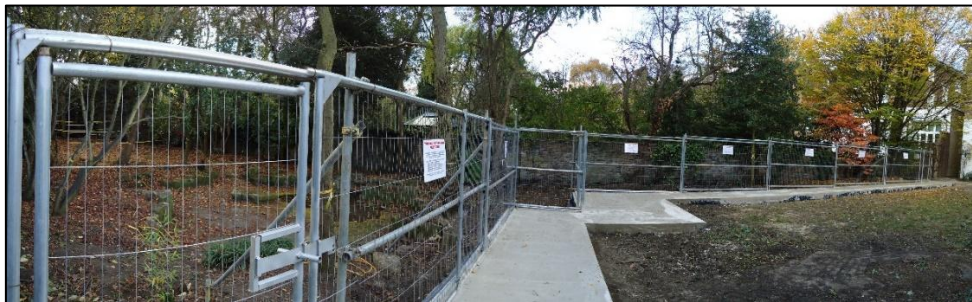
Figure 4. Photograph to illustrate installed protective fencing.
