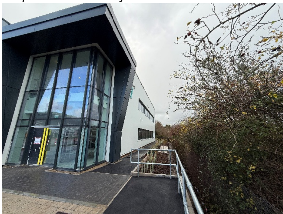
Image 6: Looking along the south elevation of the instructional unit.
