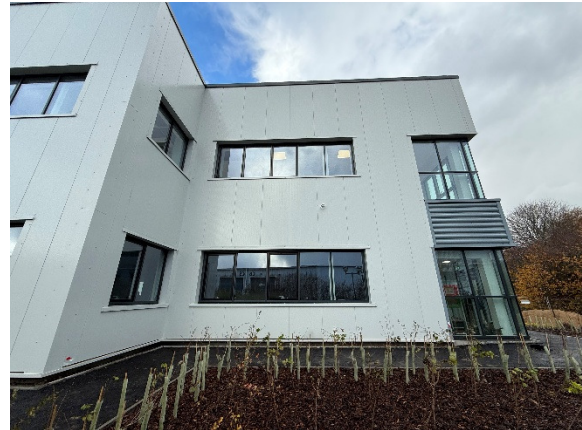
Image 5: Looking north at the setback section (escape stairwell) to the south elevation.
