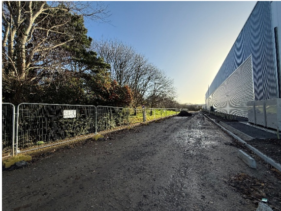
Image 4: looking south along unit 6 & 7 east elevation and existing planting, bund and newly planted beds to soften elevational treatment.
