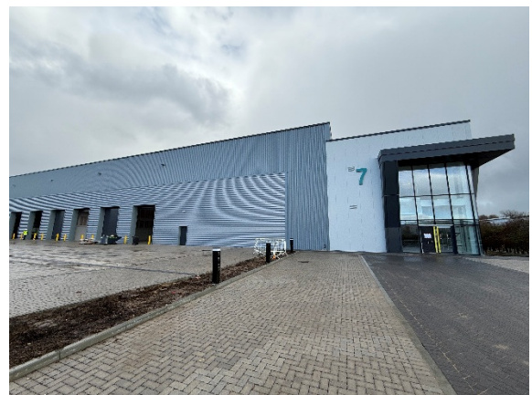
Image 7: Looking at the west elevation at the main entrance and loading bays.
