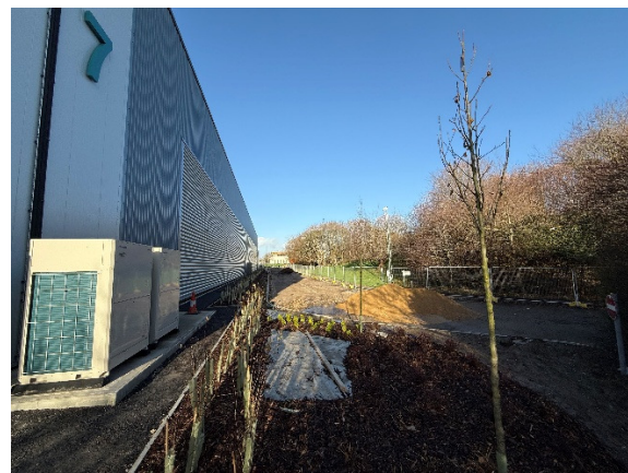
Image 3: View of east elevation at location of proposed 11 window installations, five at ground floor level and six at first floor level.
