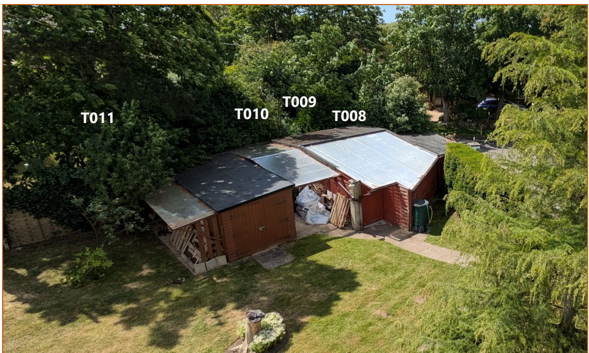
Image 5: The existing sheds sit over a concrete subbase which can be utilised for the carport and parking bay
