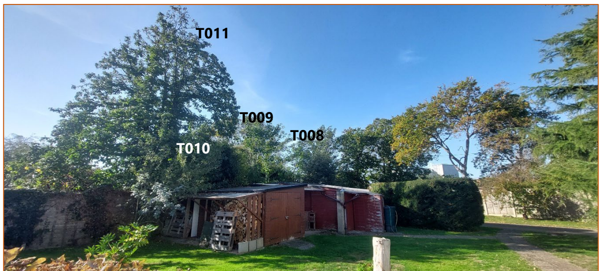
Image 3: Low branches from the adjacent neighbouring trees overhang the existing wooden garden sheds
