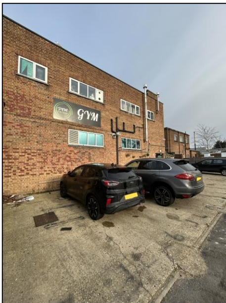
Photograph 1: Site rear forecourt
