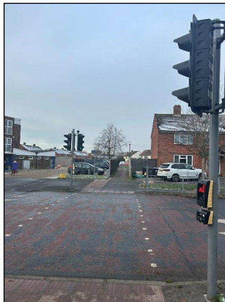
Photograph 12: Toucan Crossing on Dunsbury Way
