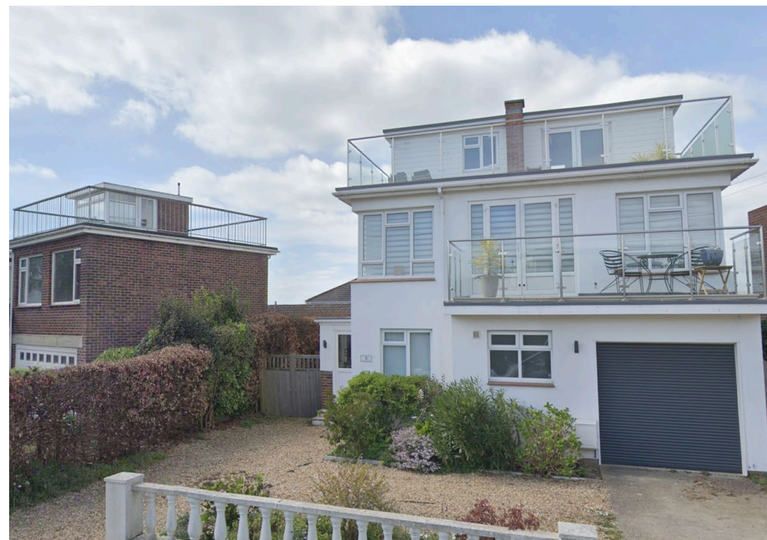
1 & 5 Wittering Road – Typical brick 2-storey dwelling and altered / extended neighbouring dwellings
