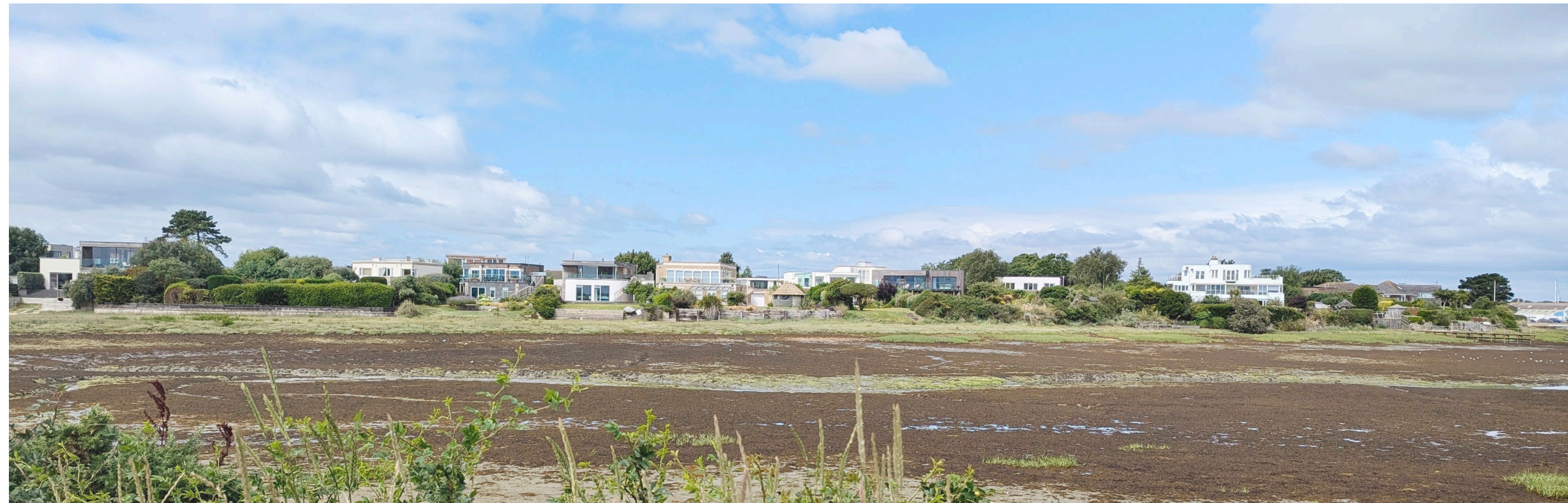
Rear view of 2 - 26 Wittering Road
