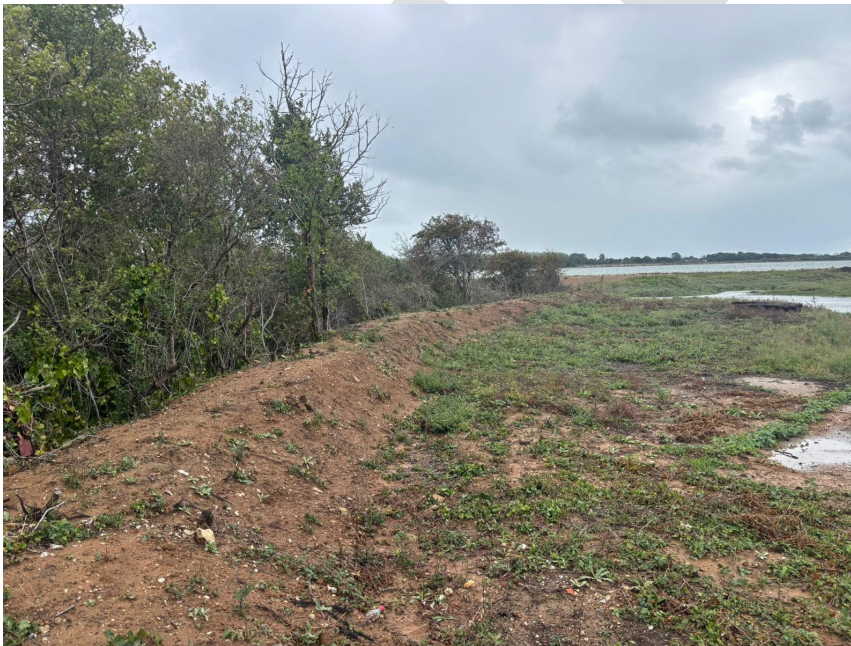
Figure 8. Disturbed bare ground and ruderal vegetation colonising on the bank recently maintained as part of a previous permission with Blackthorn scattered scrub to the southeast
