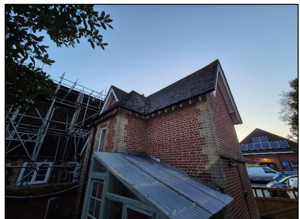
Photo 10: Well bedded hip tiles.
