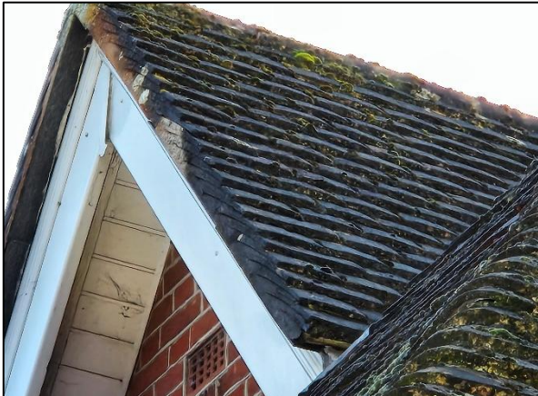
Photo 15: Well fitted soffits and barge boards.
