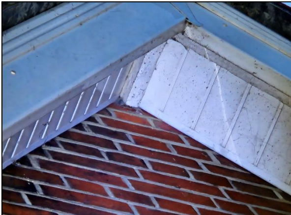
Photo 15: Well fitted soffits and barge boards.
