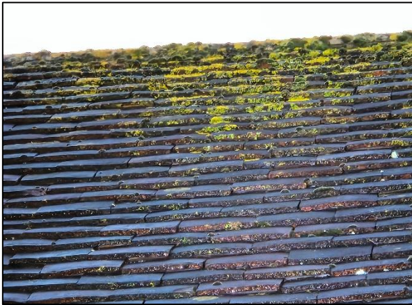
Photo 11: East facing roof tiles.
