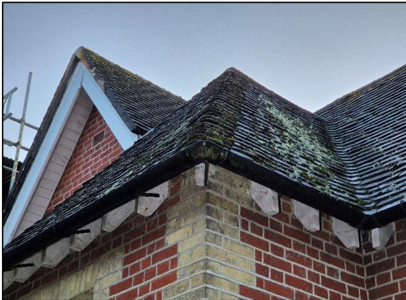
Photo 9: Roof tiles on north and east elevations.
