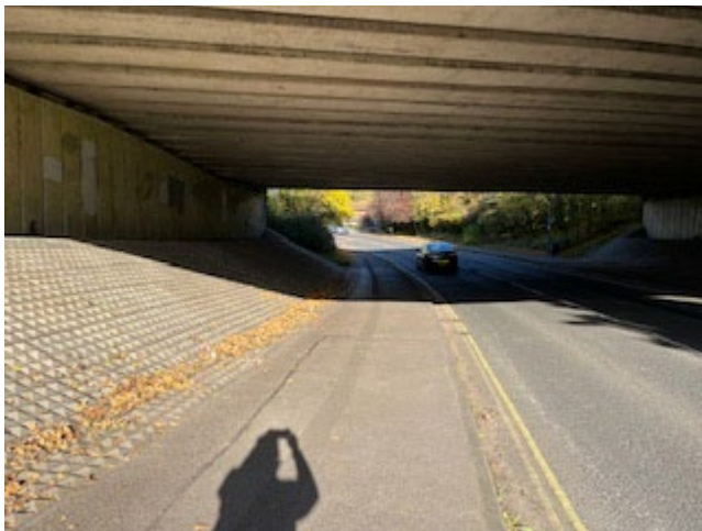
Figure 1: Crossing point after underpass.
