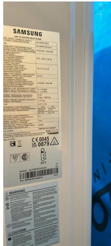
Photo 2: ASHP Spec plate (unit 1)
