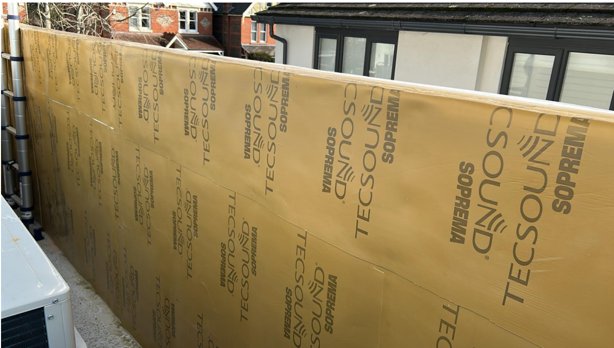
Photo 6: Inner face of barrier (Techsound in place)
