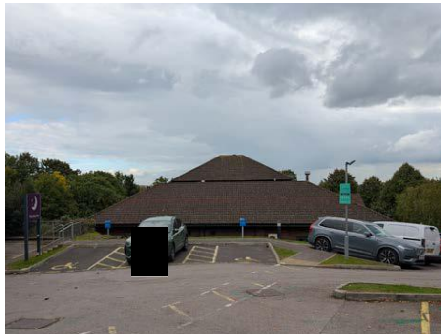
1) Site Entrance looking South - Existing
