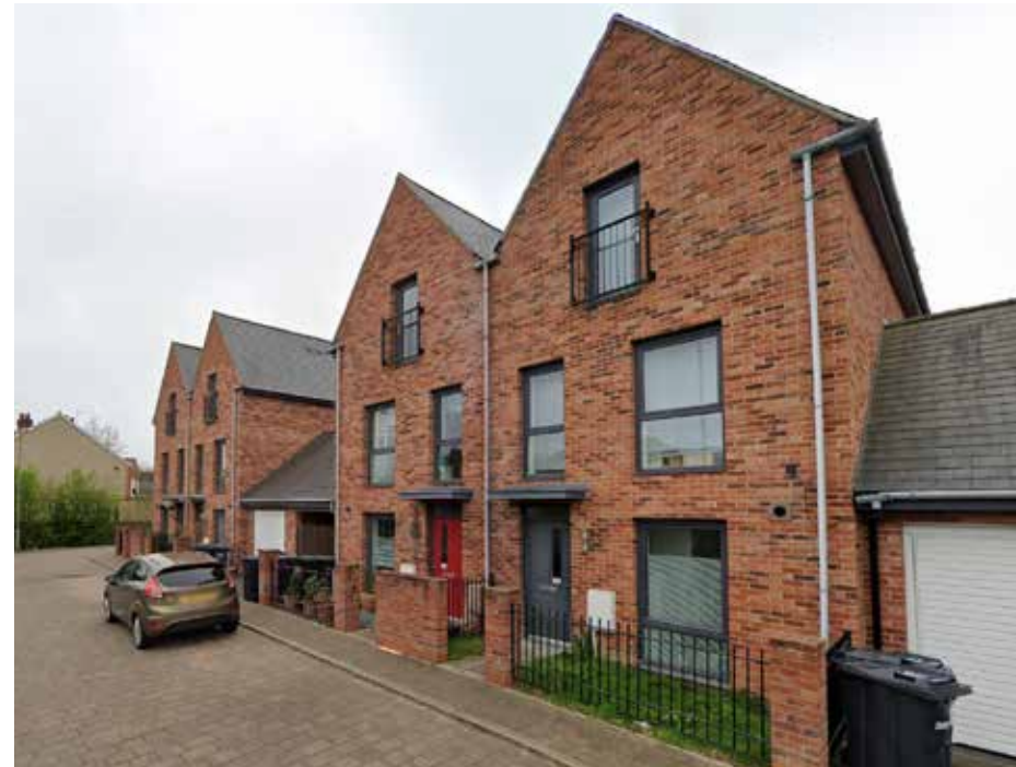
Three-Storey Semi-Detached Houses with Sawtooth Roof
