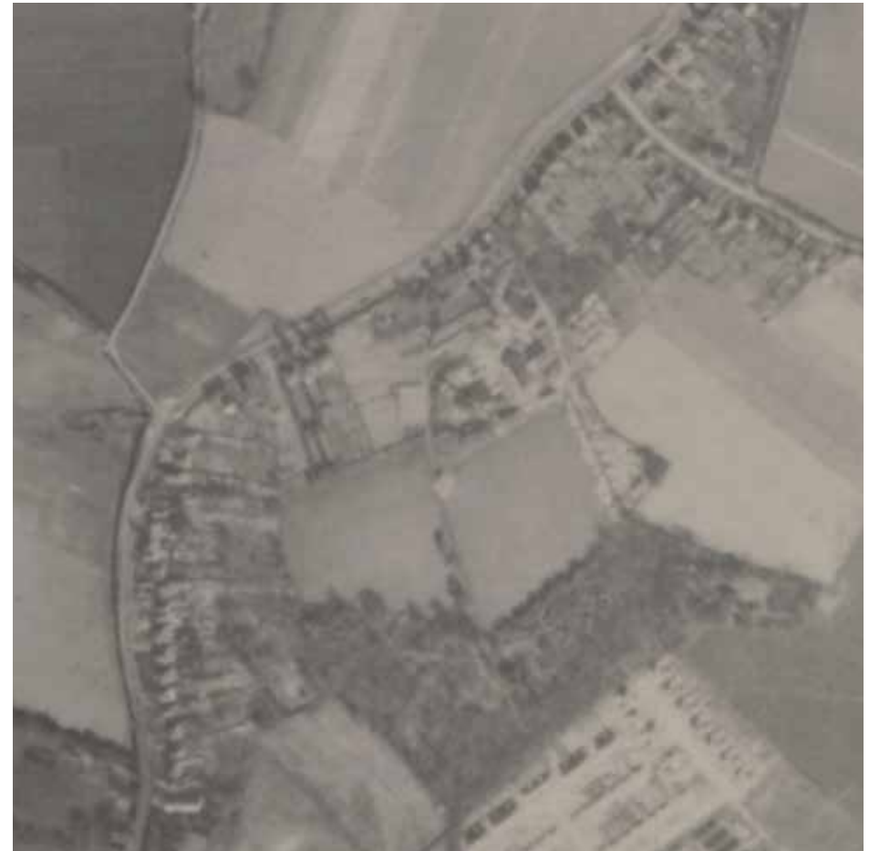
Aerial photograph from circa 1945 showing J.F Goodwillie Ltd on site
