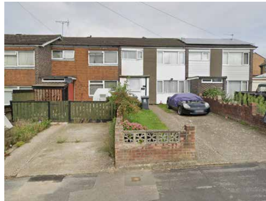
Terraced Houses on Corbett Road featuring tandem-parking and gardens to the front.
