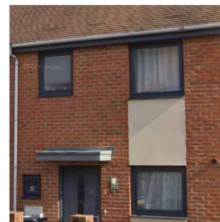
Contrast Panels Linking Windows
