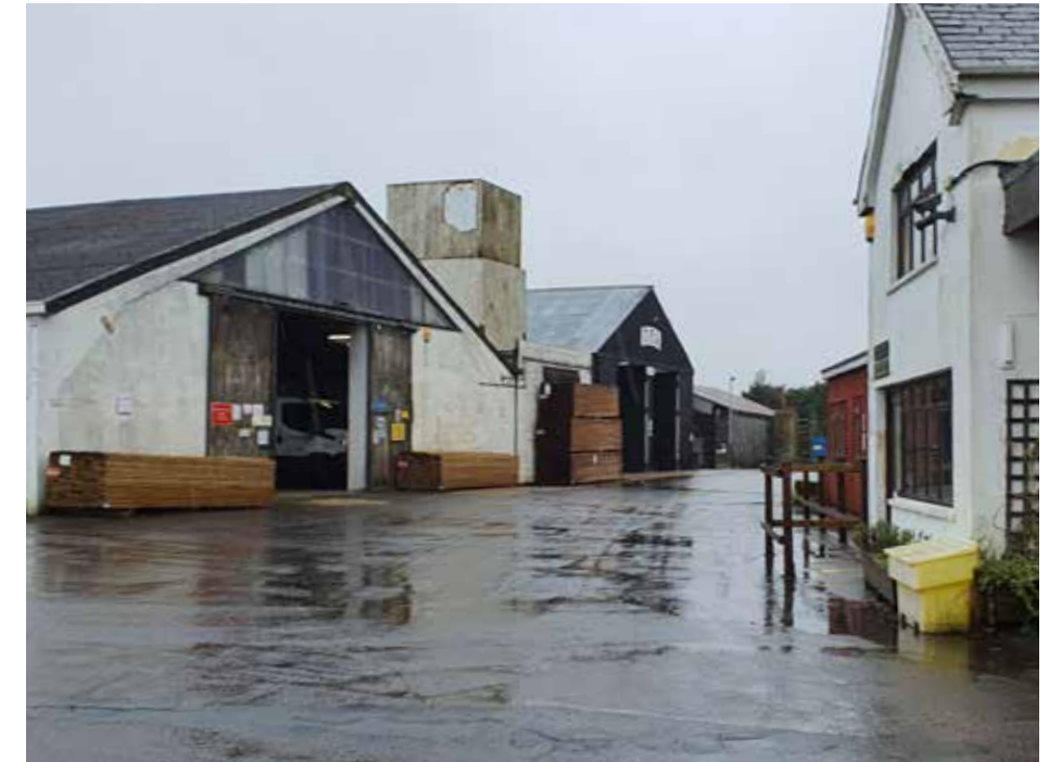
Large timber warehouses connected by a circa 5m tall roofed building.
