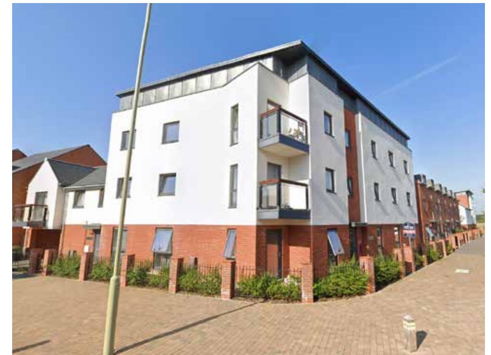
Corner-Turning Block of Flats
