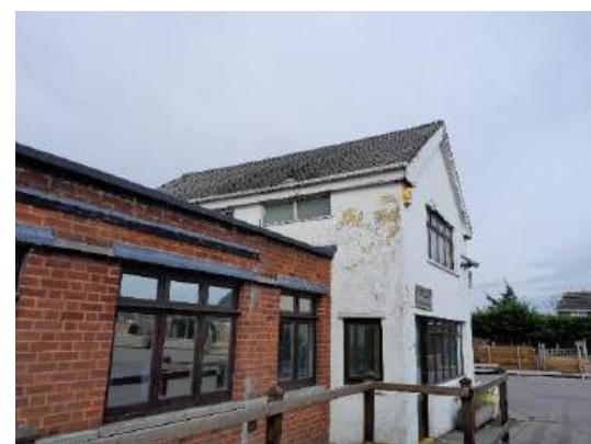
Photo 6: B4, south-western aspect
