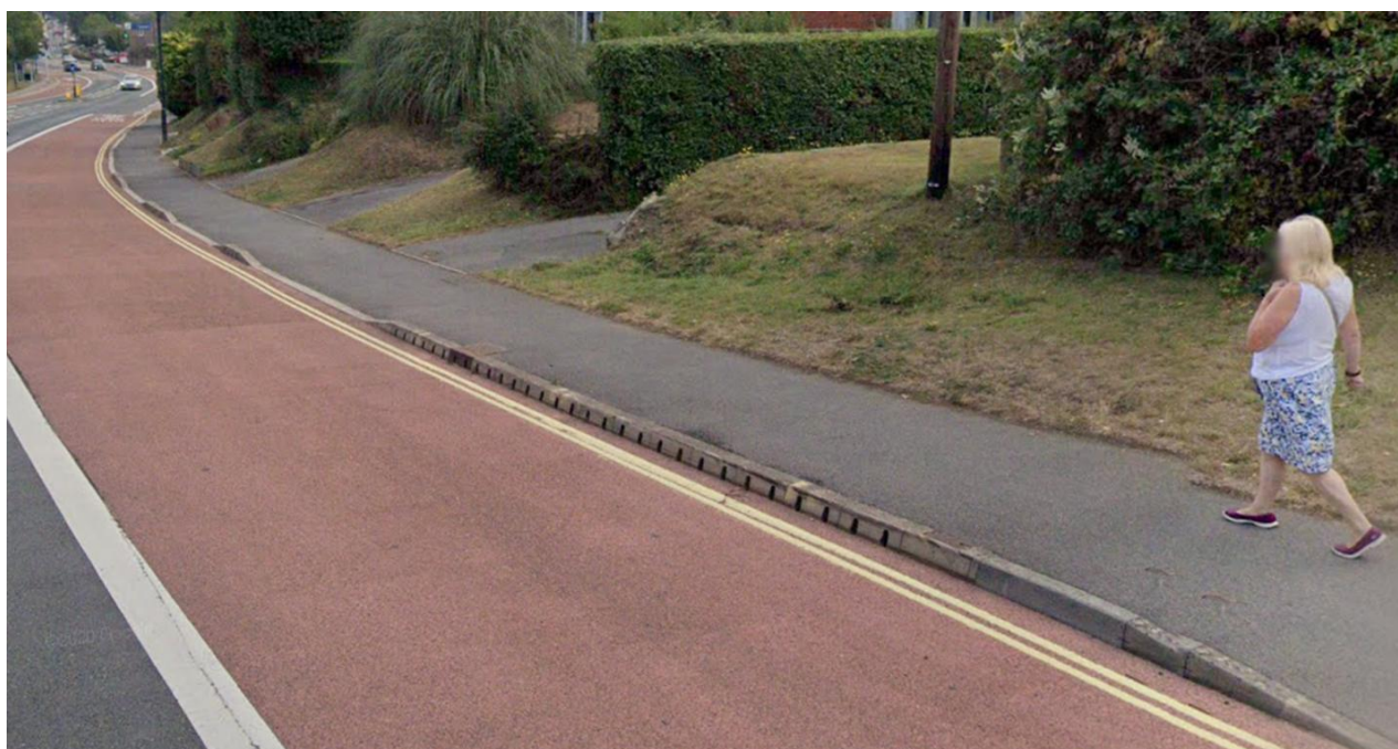
Figure 2.5: Existing Footway Flanking the A3 London Road
