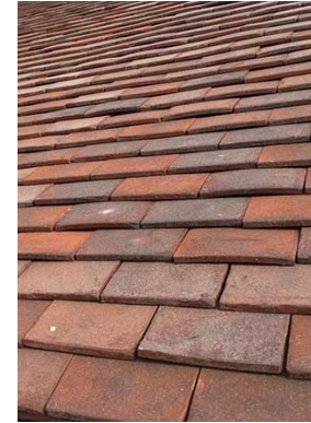
Red Tile Roof
