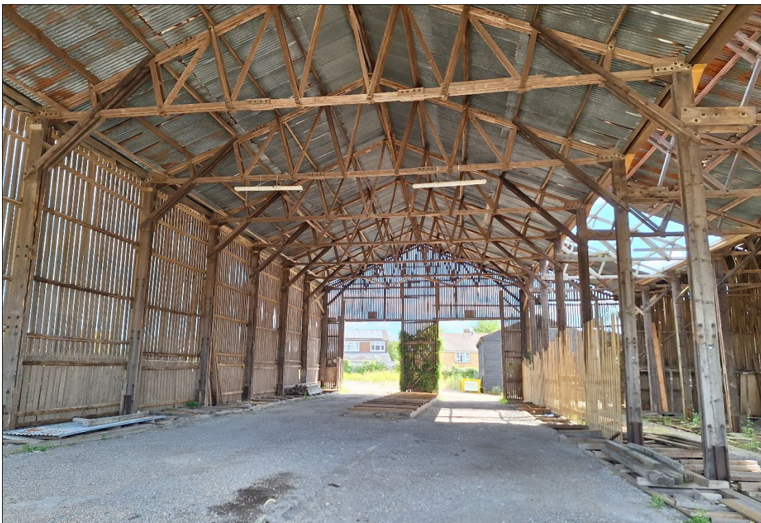
Photo 2: Within large timber storage sheds in the south-east of the Site
