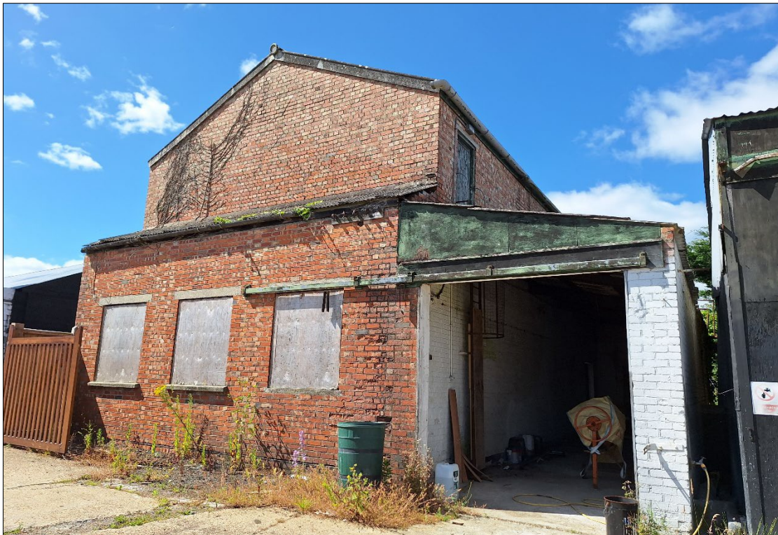
Photo 4: Former kiln building in central part of the Site
