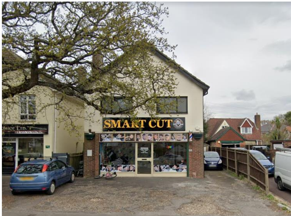
Fig. 1: View of existing building.
