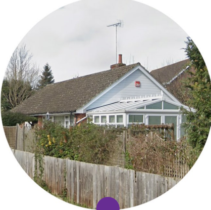
20 LOWER ROAD WHITE WEATHERBOARD
