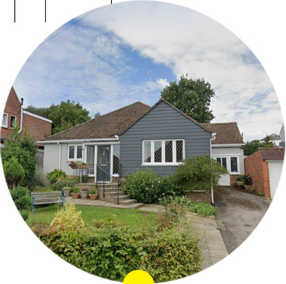
25 LODGE ROAD GREY WEATHERBOARD & LIGHT RENDER
