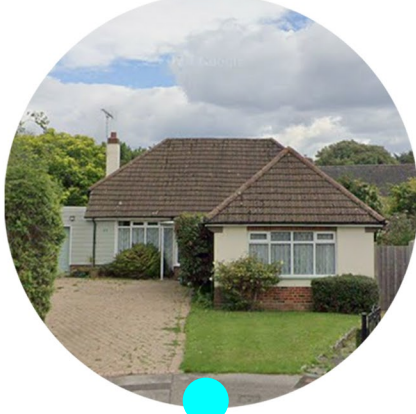
26 LODGE ROAD LIGHT WEATHERBOARD & CREAM RENDER
