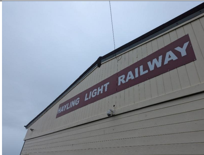
Figure 10. The eastern elevation of the Hayling Light Railway Depot (photo taken November 2025).
