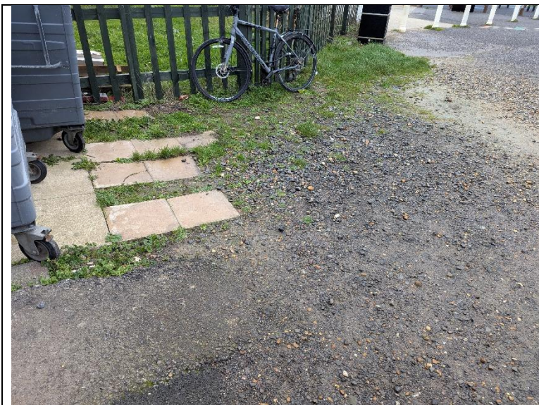
Figure 1. The small section of unsealed surface within the site boundary (photo taken November 2025).
