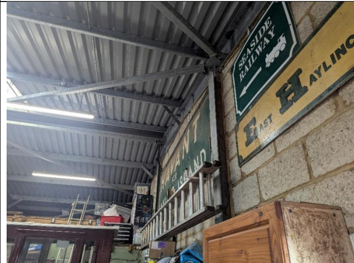
Figure 11. The internal wall of the eastern elevation of the Hayling Light Railway Depot (photo taken November 2025).
