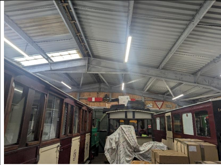
Figure 9. The internal space of the Hayling Light Railway Depot (photo taken November 2025).
