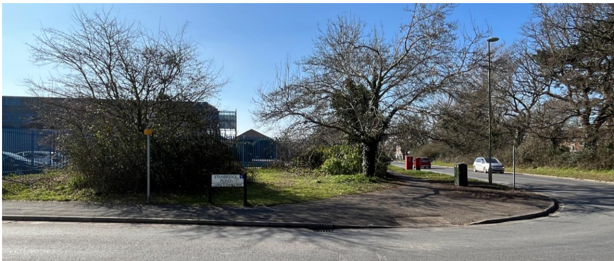
Figure 9 Streetscene Photo of the Buildings Location on the New Lane/Stanbridge Road Junction
