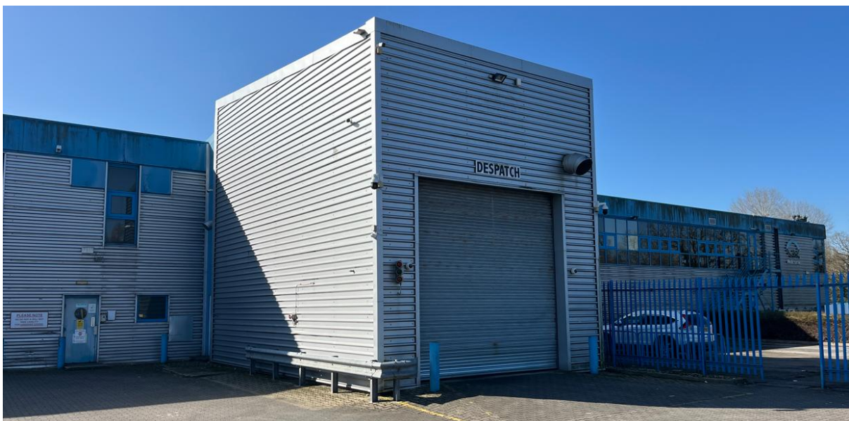
Figure 7 Loading Bay on Buildings North Elevation
