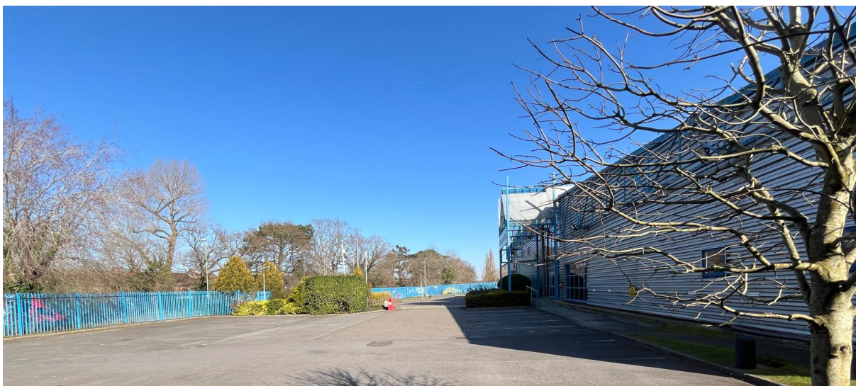
Figure 4 View North Across Parking Area to West of the Building
