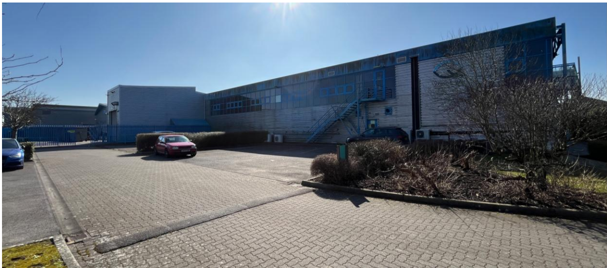
Figure 6 View from North-West Towards Buildings North Elevation
