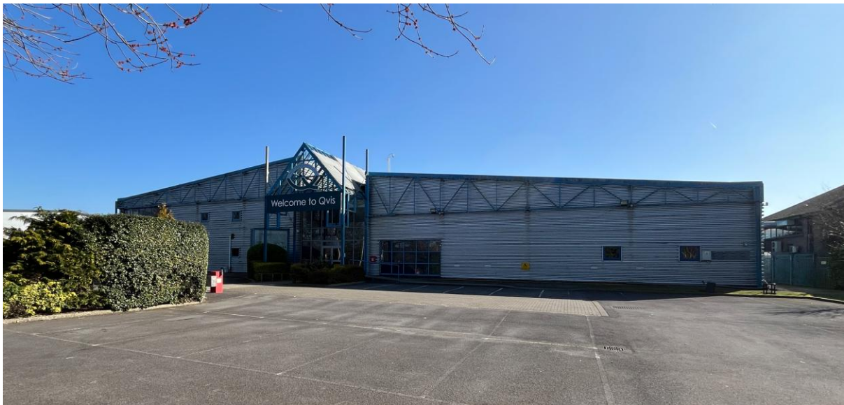
Figure 3 View of the Buildings west Elevation from Boundary Fence
