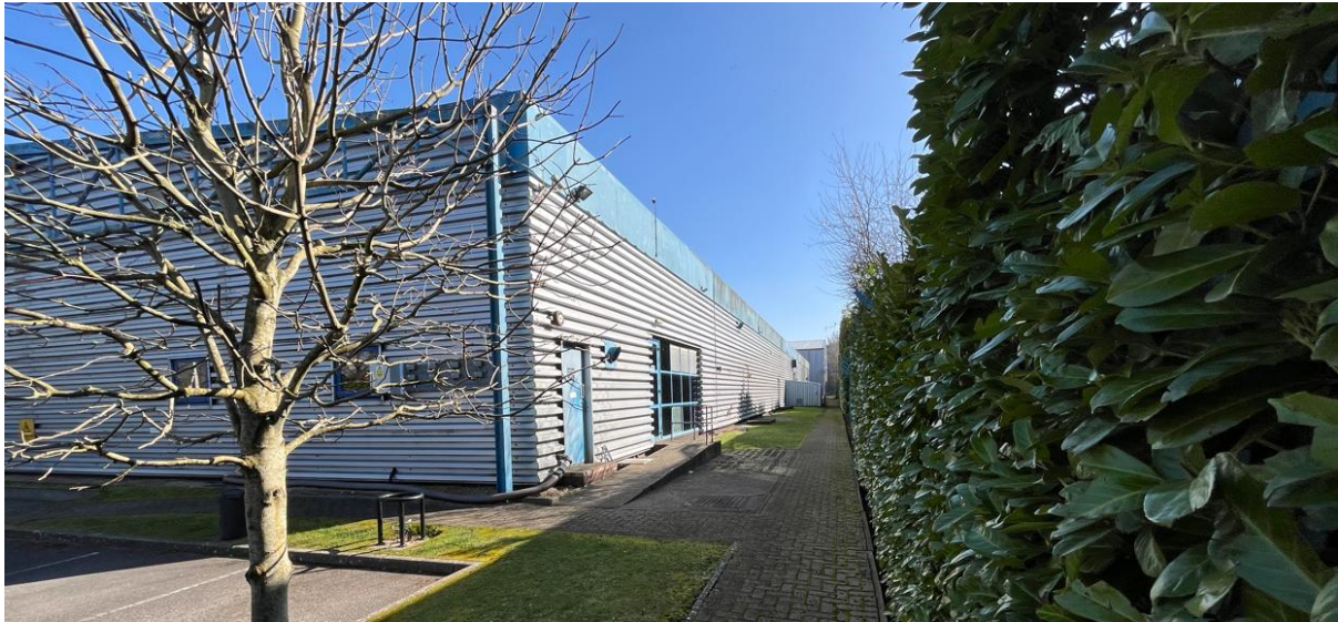
Figure 5 View East Showing the Buildings South Elevation
