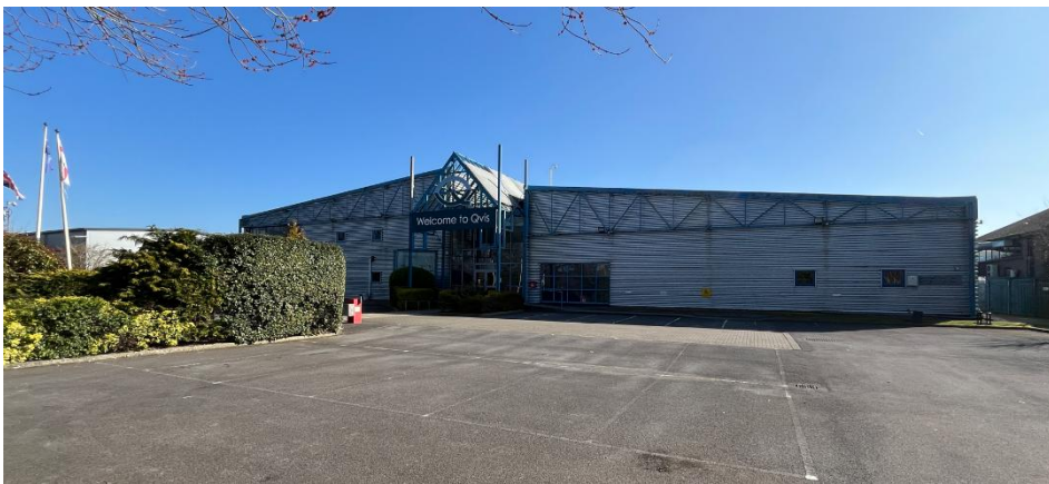
Figure 1 36, New Lane, Havant – West Elevation
