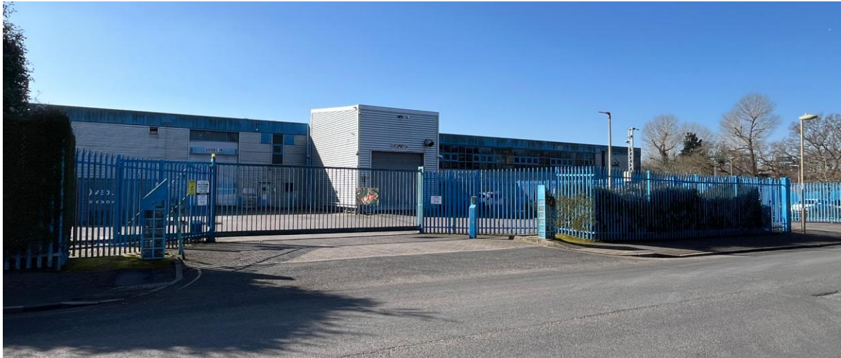
Figure 8 Streetscene Photo taken From North Side of Stanbridge Road towards Building
