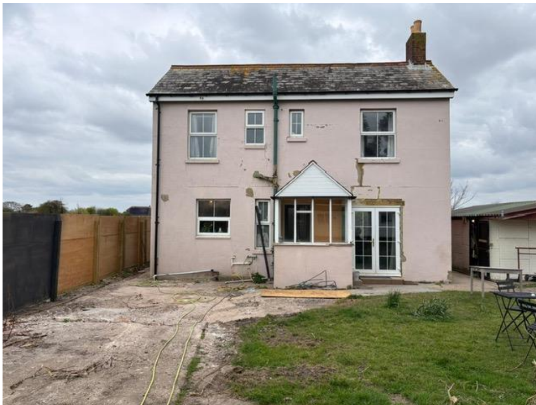
The rear elevation will lose the rear porch which is of poor quality, the existing windows are low quality upvc in a range of styles this elevation is of little architectural or historic significance
