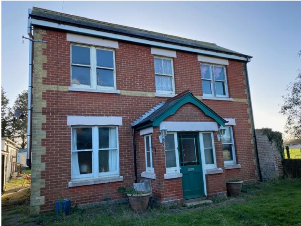
The front Elevation including sash windows, stone lintels stone cills and corner quoin stones will remain unaffected by the application.
