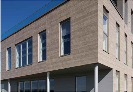
New external cladding. Rockpanel or similar (suggested pale / neutral colour in stone or wood finish).
