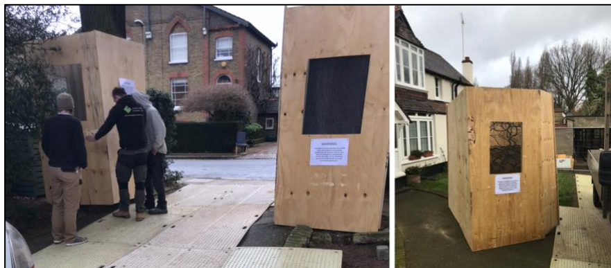
Image 6: Examples of trunk protection hoarding. (NOT USED ON THIS SITE)
