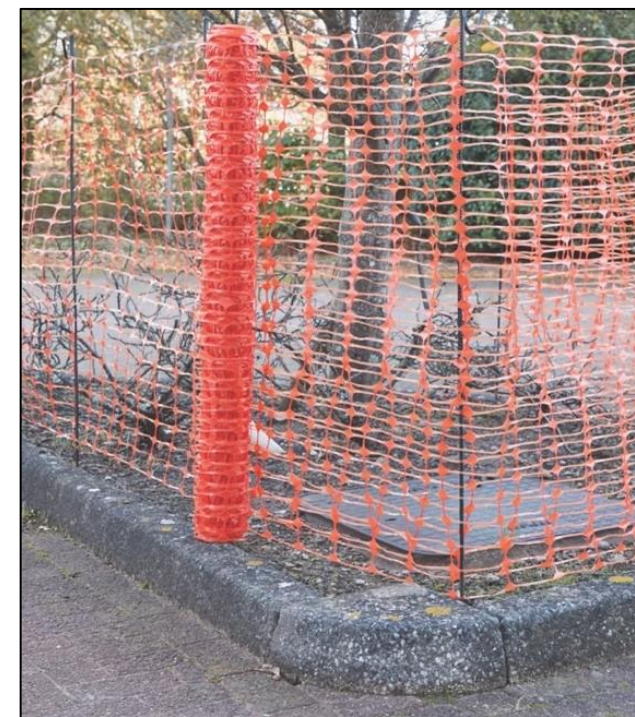
Image 3: Showing orange netlon fencing supporting by road pins. (NOT USED ON THIS SITE)
