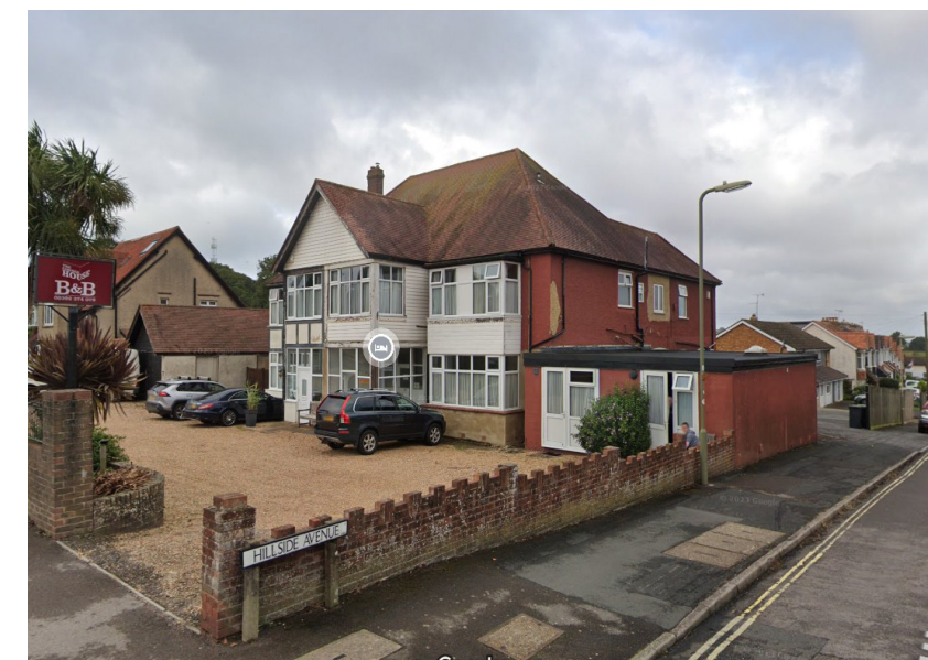
Corner View at junction of London Road and Hillside Avenue
