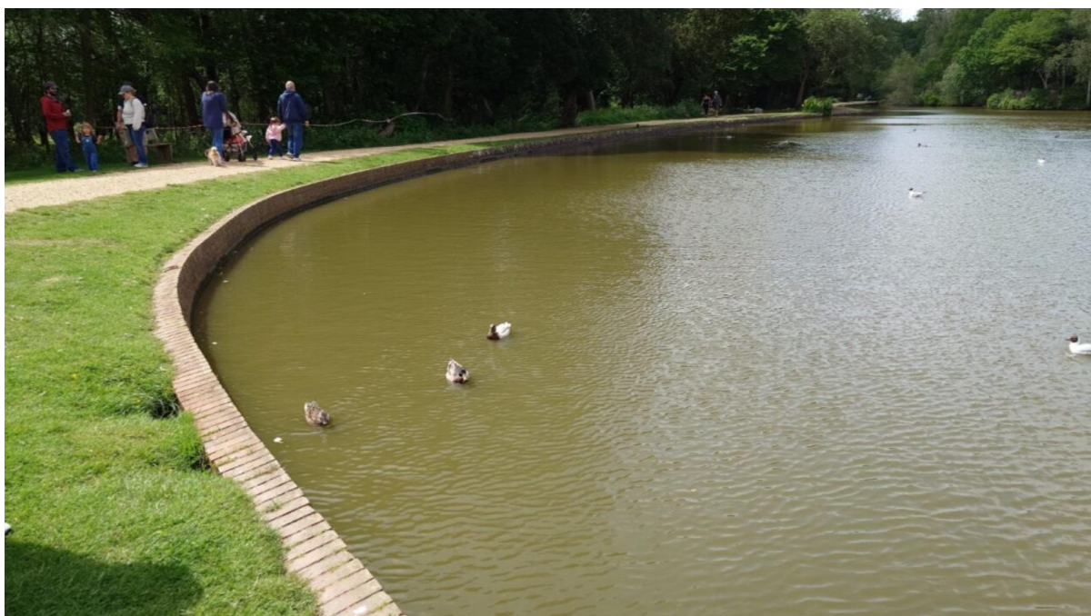
Photo 1: Typical form of the lake wall on its southern boundary
