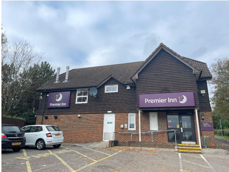
Entrance to the existing hotel building
