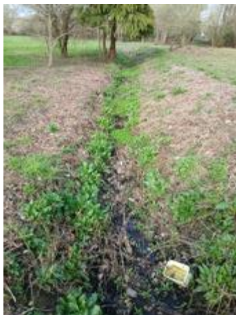
Photo 23: A view facing north along drain D2.
