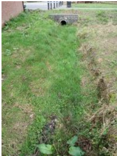
Photo 21: A vegetated section of drain D1 and a culvert.
