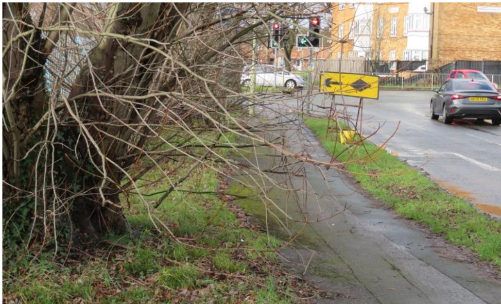
Photo 2: Looking west along Barton Road towards Petersfield Road junction
