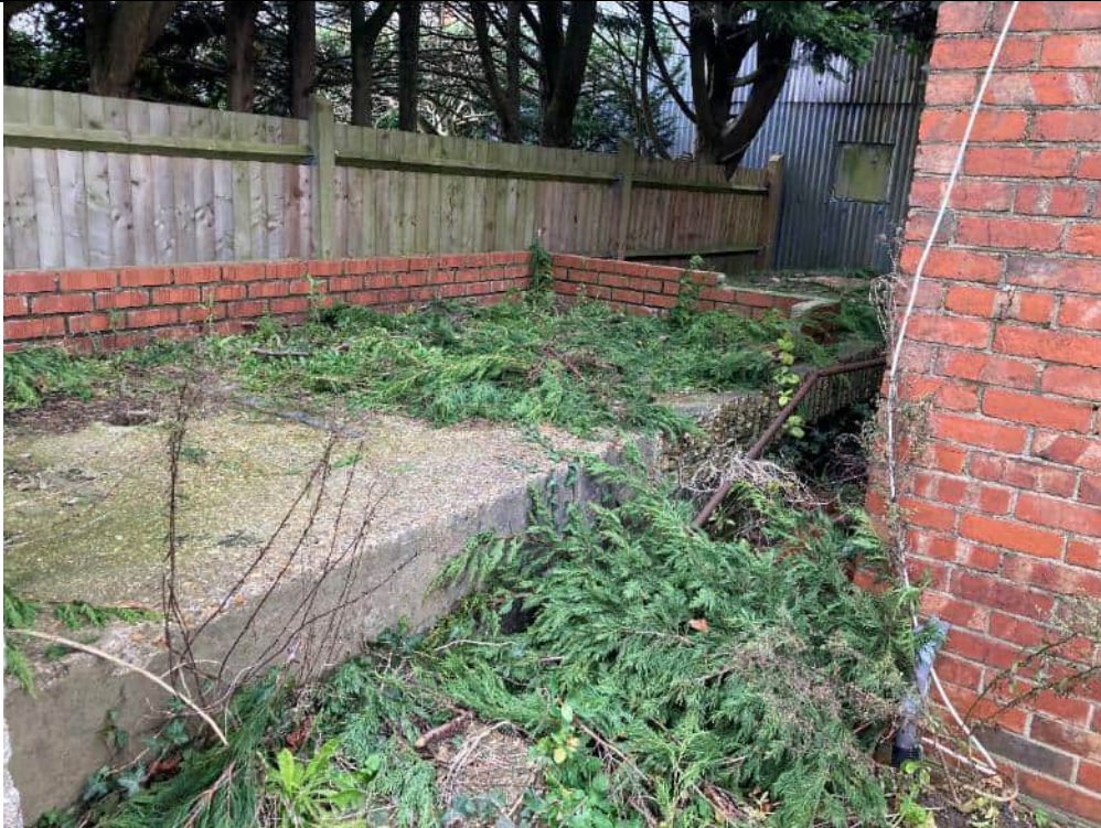
Photograph 11 – Outside construct of the underground bunker – December 2024
