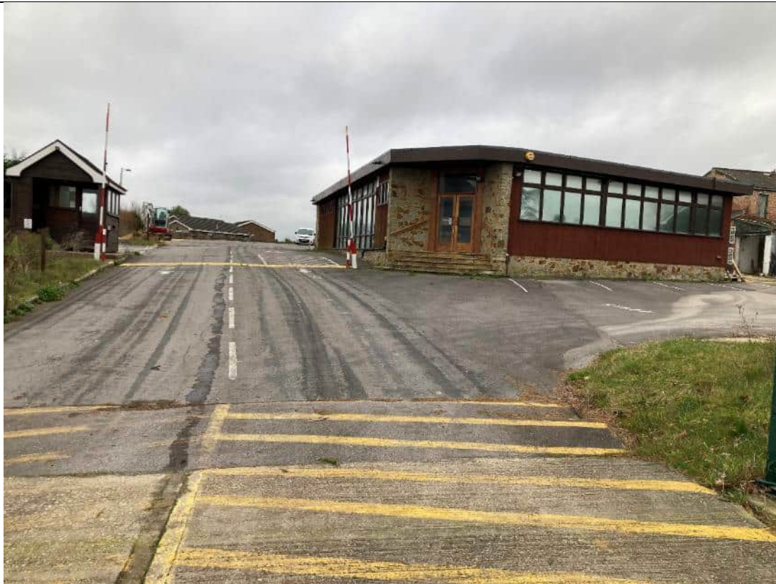
Photograph 1 – Entrance to site from London Road (facing south) – December 2024
