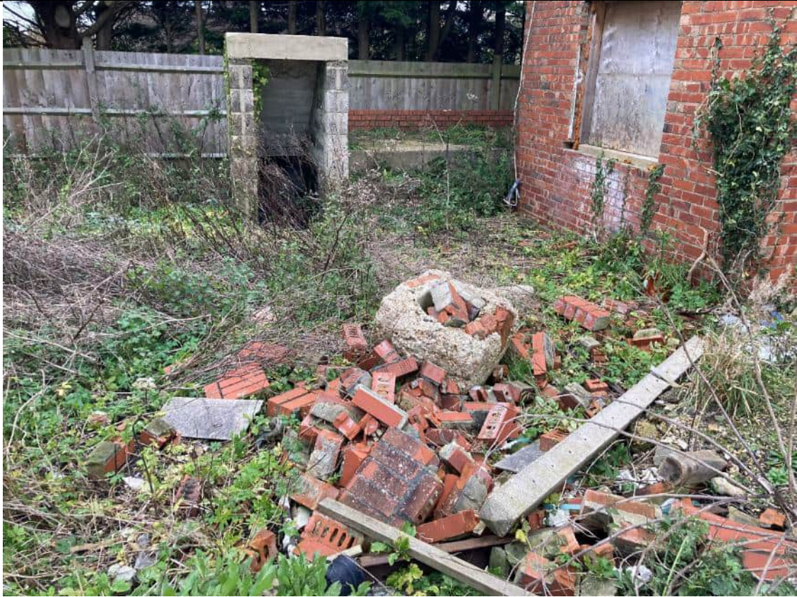
Photograph 9 – Entrance to the underground bunker – December 2024
