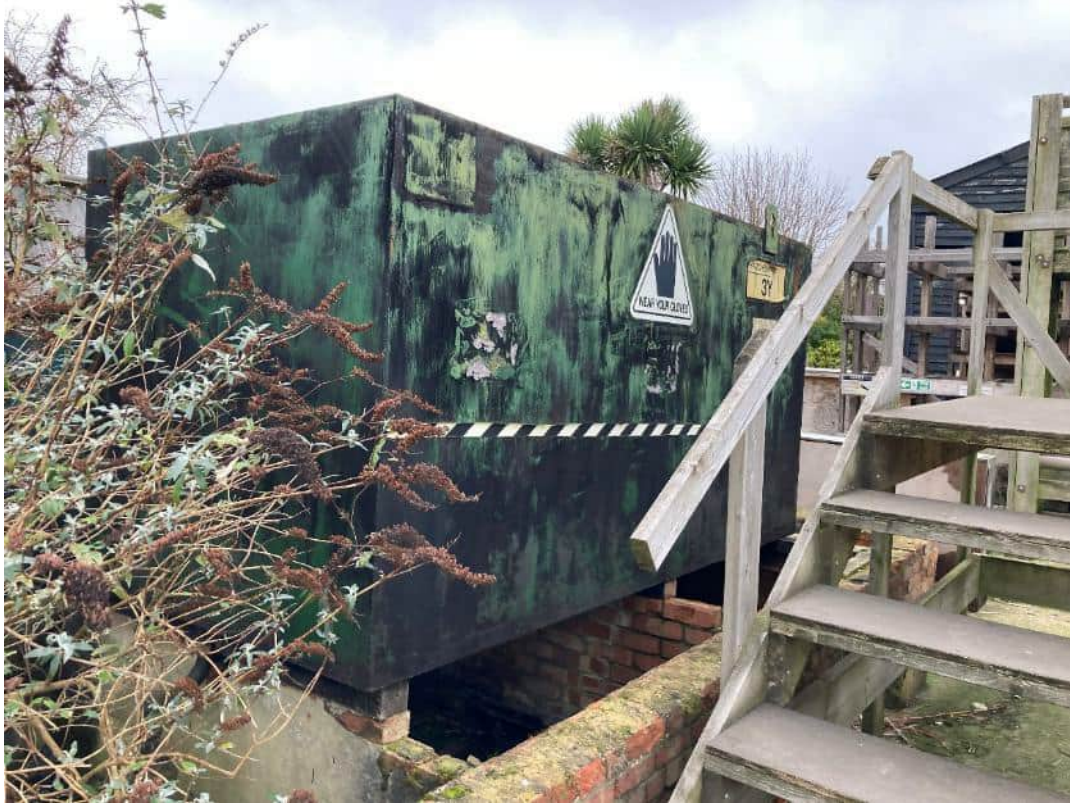
Photograph 13 – Storage tank in the northwest of the site – December 2024
