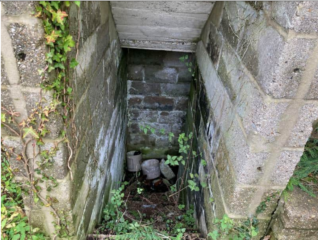
Photograph 10 – Entrance to the underground bunker – December 2024
