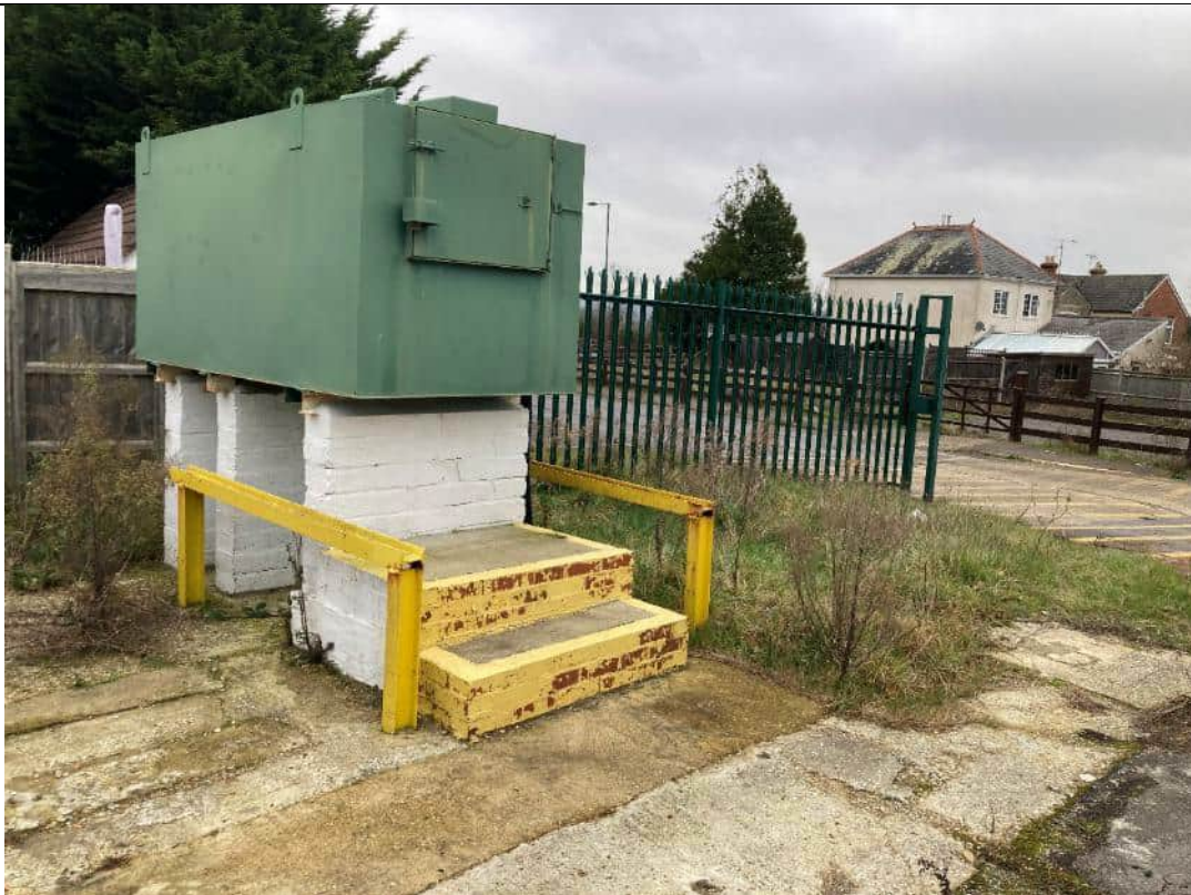
Photograph 12 – Storage tank in the north of the site – December 2024
