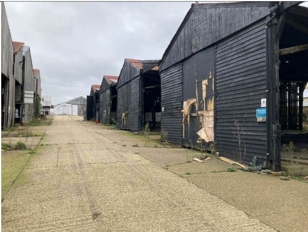
Photograph 6 – Overview of the eastern area of the site (facing north) – December 2024
