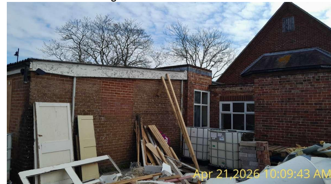
Showing the southern elevation of B1.
