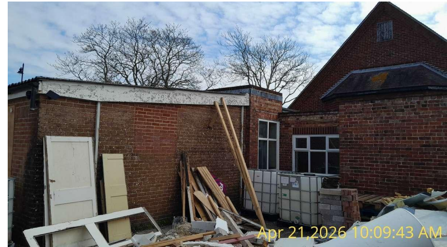
Photo 2: Showing the southern elevation of B1.
