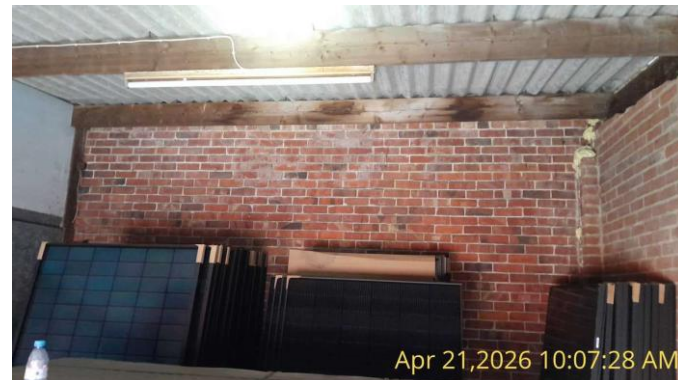
Showing the southernmost room within the garage, looking east.
