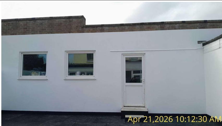
Photo 3: Showing the northern elevation of B1.
