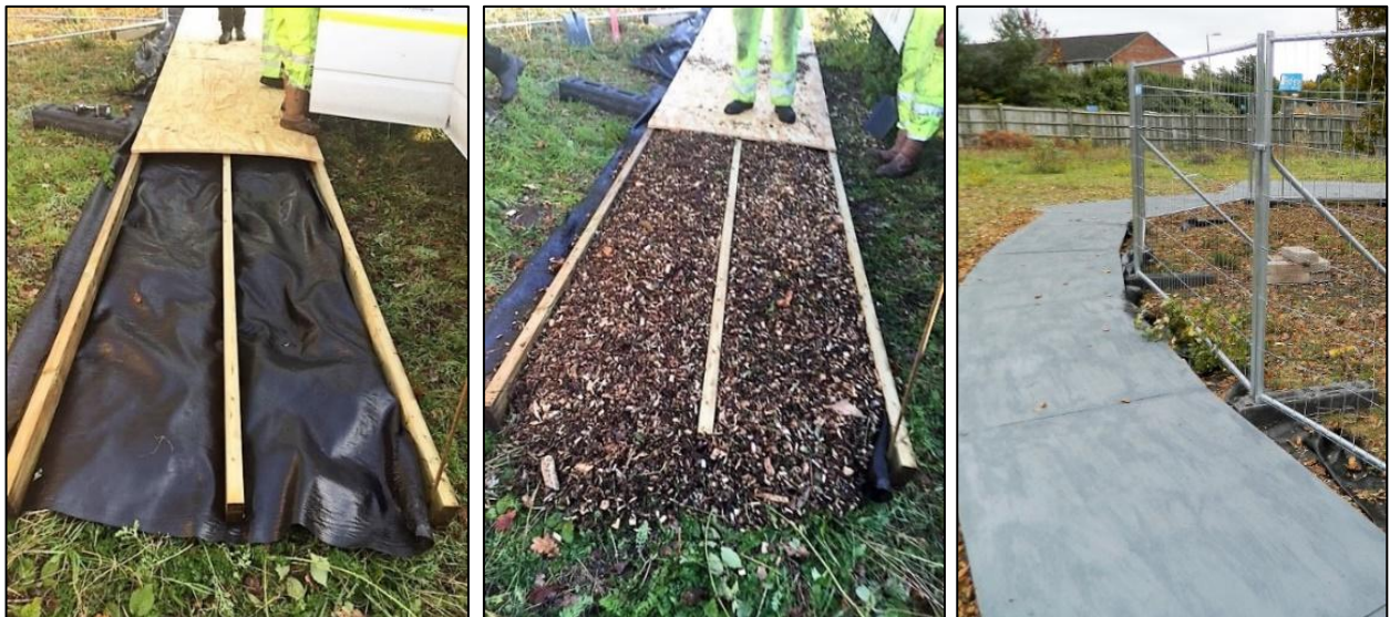
Figure 7. Plywood sheeting supported by timber bearers with woodchip infill used as ground protection for parts of the RPA outside fencing.
