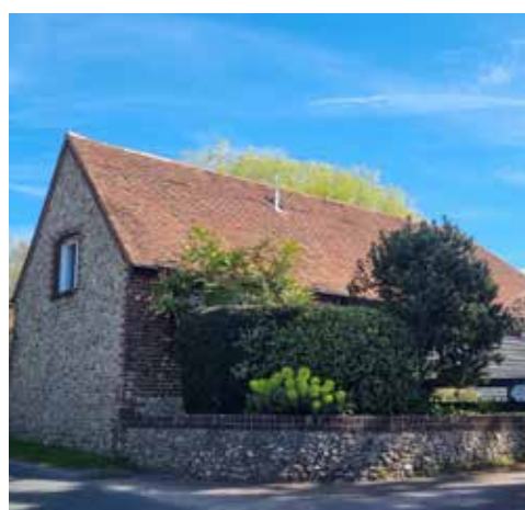
House along Eastleigh Road showing flint, red brick and weatherboard
