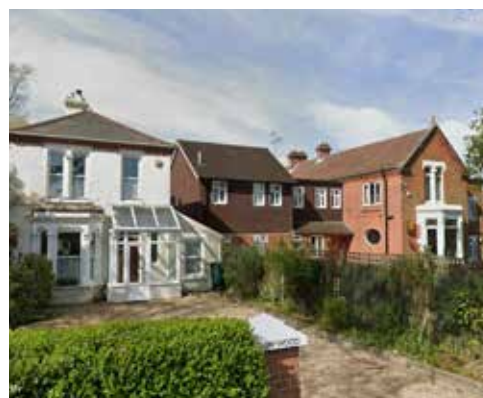
Horndean Road - Detached houses with bespoke architectural detailing
