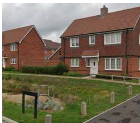
Normandy Way - Use of hanging tiles
