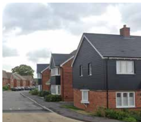
Normandy Way - Use of red brick and weatherboarding
