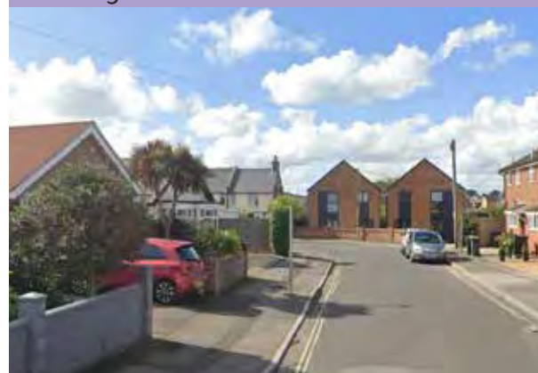
St James Road - building heights vary between 1 and 2 storeys
