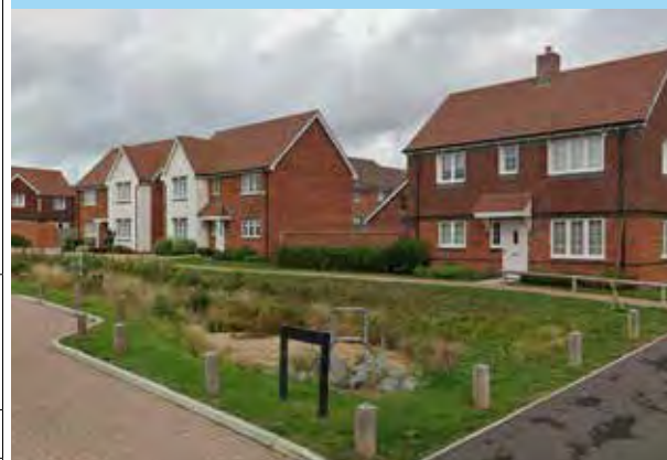
Normandy Way - Use of hanging tiles
