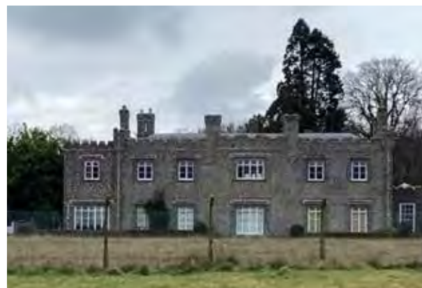
Southleigh Park House - Historic landmark building overlooking Southleigh Park
