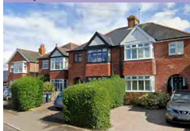
St James Road - Consistent architectural detailing and material choice
