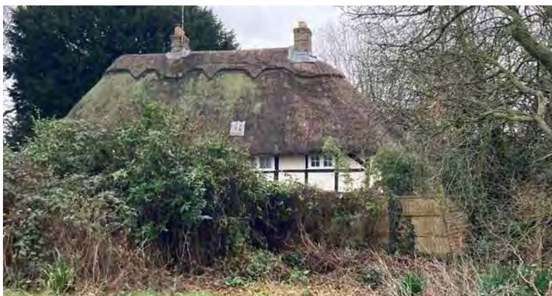
Nos. 1 and 2 Eastleigh Road viewed from the west (No.24703)
