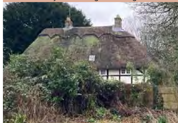
Thatched roof house with generous front garden and mature vegetation
