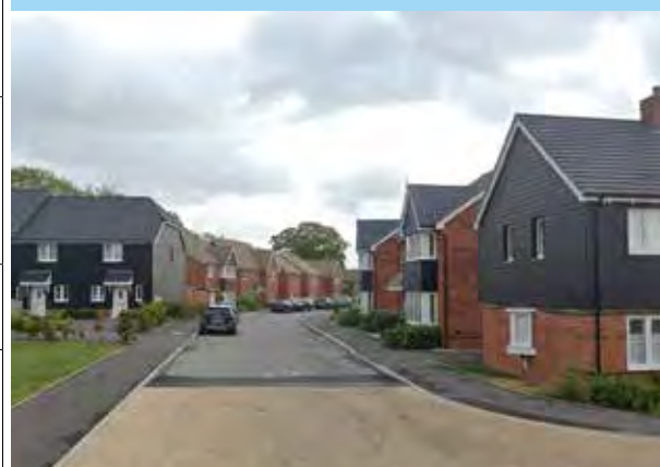
Normandy Way - Use of red brick and weatherboarding
