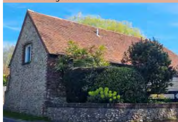
House along Eastleigh Road showing flint, red brick and weatherboard
