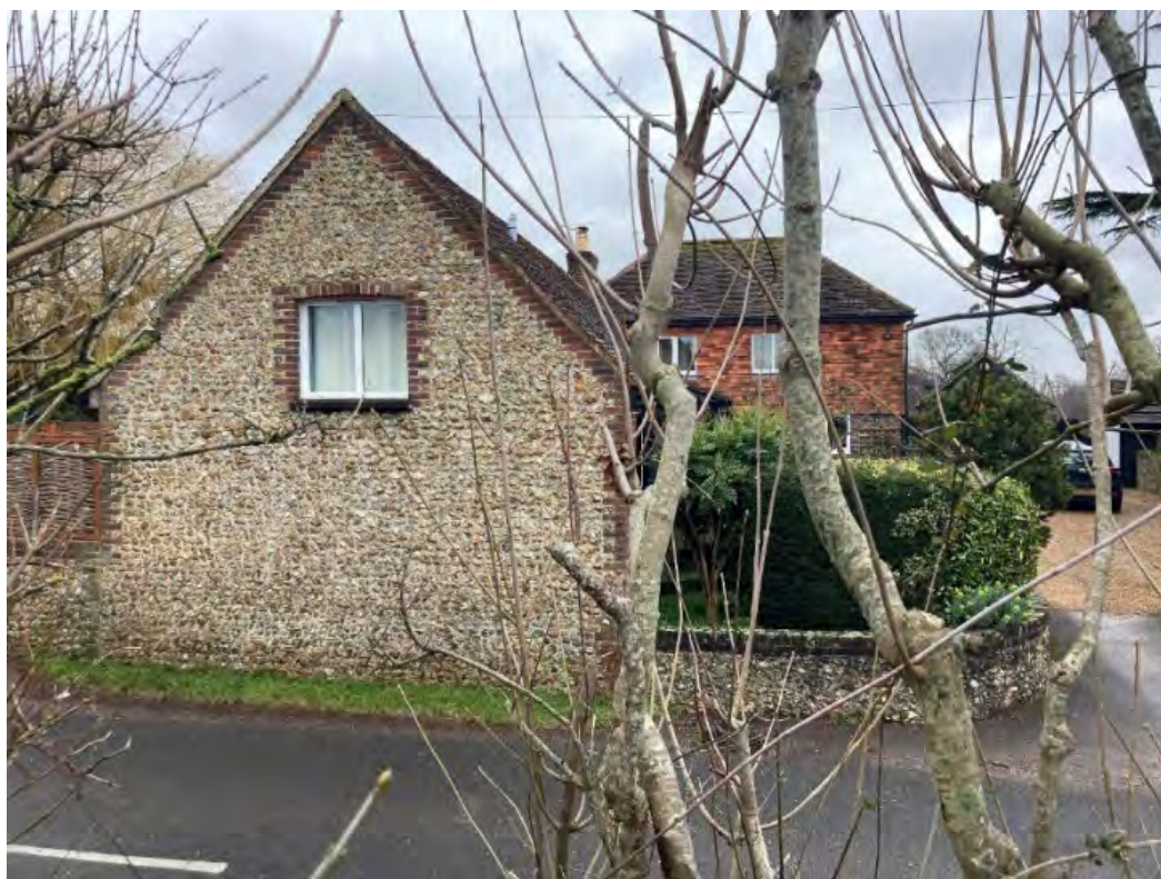
Figure 12: West elevation of Home Farm Barn.
