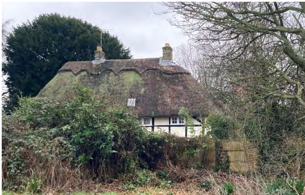
Figure 7: Nos. 1 and 2 Eastleigh Road viewed from the west.
