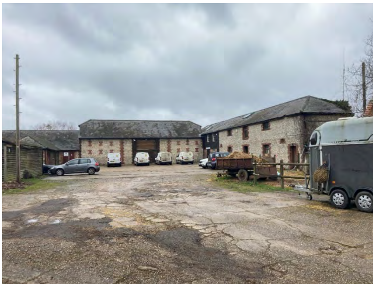
Figure 14: The north and west ranges of Southleigh Farm arranged around the farmyard.
