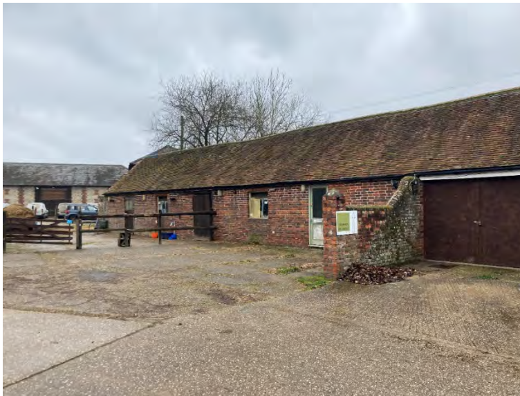
Figure 13: The south elevation of the northeast range.
