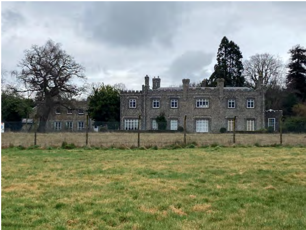
Figure 9: The south elevation of Southleigh House.
