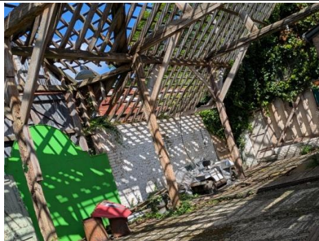
Photo 19. Internal view of B7
