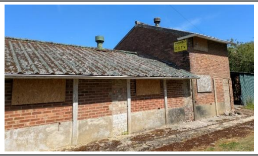
Photo 34. Southern elevation of B13
