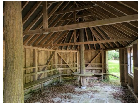
Photo 10. Internal view of B4
