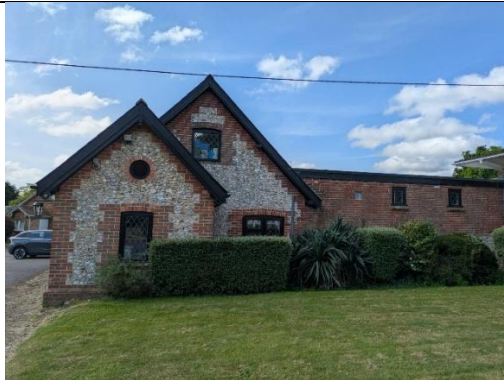
Photo 11. Northern elevation of B5
