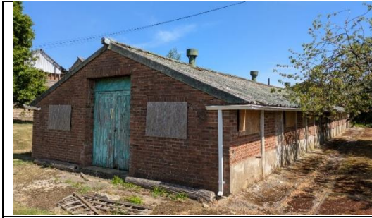
Photo 33. Western and southern elevations of B13
