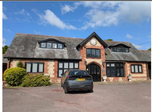
Photo 12. Eastern elevation of B5
