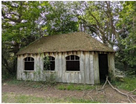
Photo 9. Eastern and northern elevations of B4
