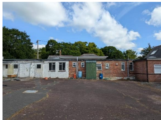
Photo 14. Southern elevation of B6
