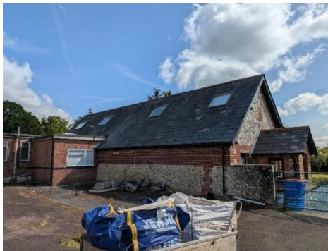
Photo 13. Western and southern elevations of B5 (right of image) and southern elevation of B6 (left of image)
