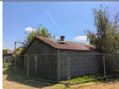
Photo 22. Northern and western elevation of B9
