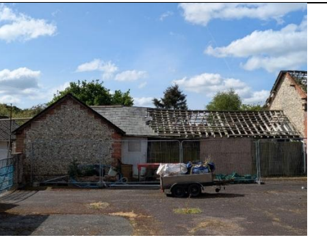
Photo 24. Northern elevation of B10
