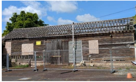
Photo 17. Eastern elevation of B7
