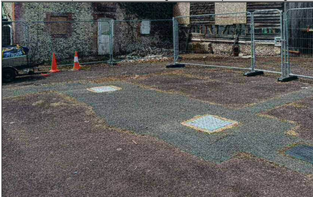
Photo 8: Drainage observed onsite.
