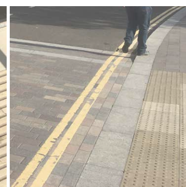
Demarcation - Kerbs of contrasting colour to pavement & road aid the partially sighted
